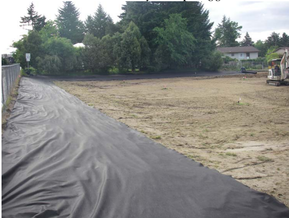
Photo D-1: Lee Elementary School placing geotextile
