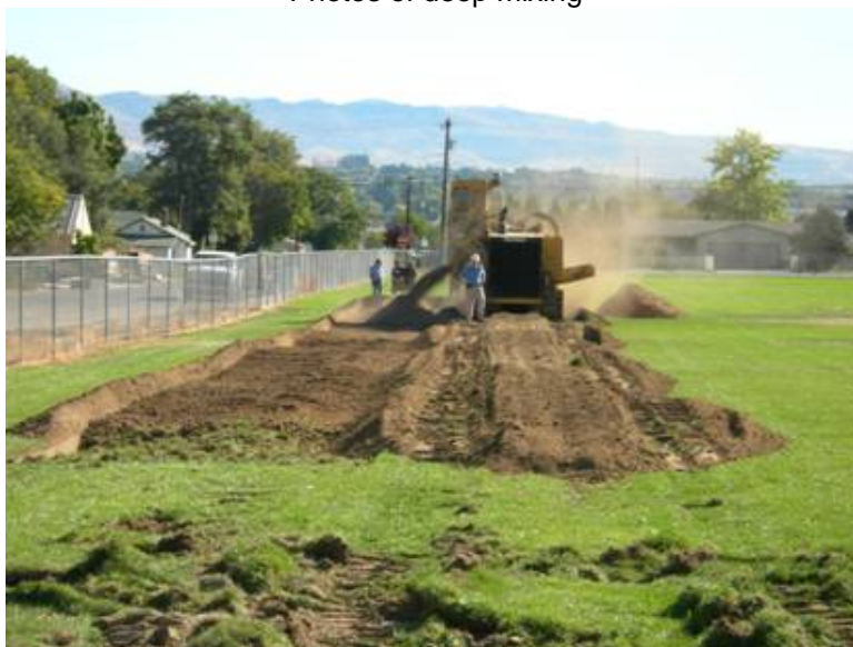
Photos of deep mixing
