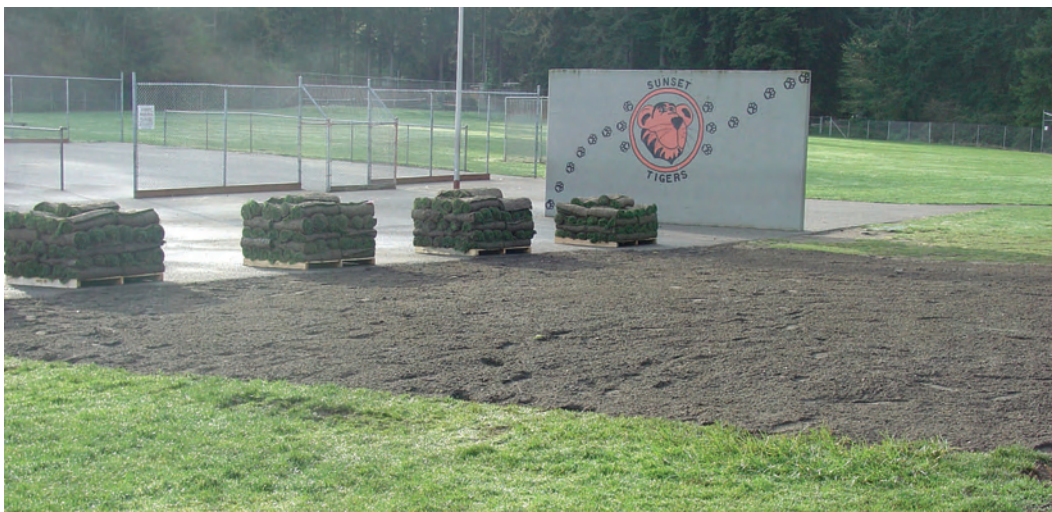
Image 6. Construction activities at Sunset Primary in the University Place School District
