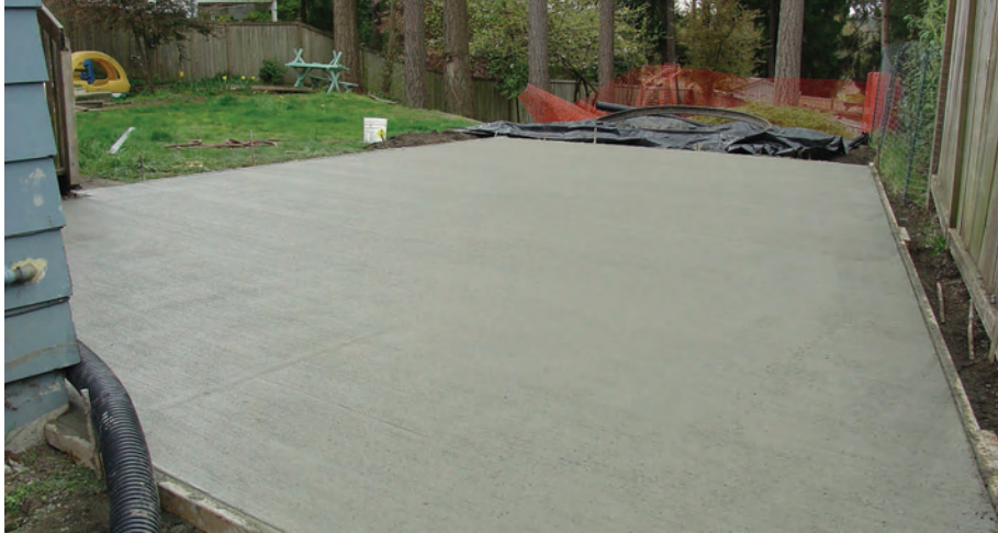
Image 3. Covering contaminated soil with concrete
