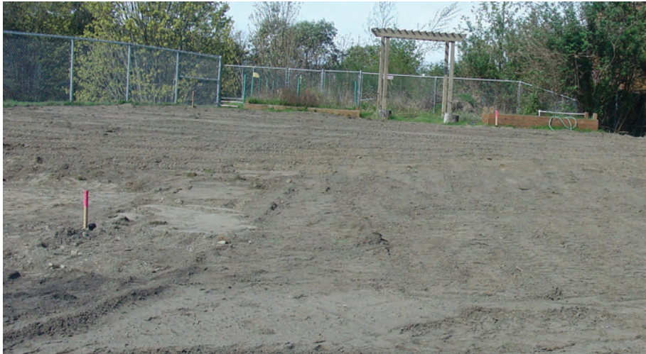
Image 4. Mixing contaminated soil with clean soil
