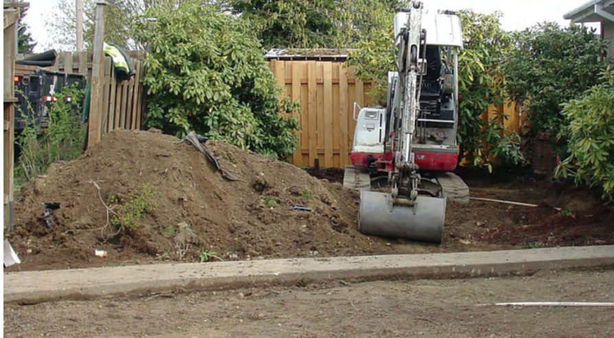
Image 1. Removal of the top six inches of contaminated soil
