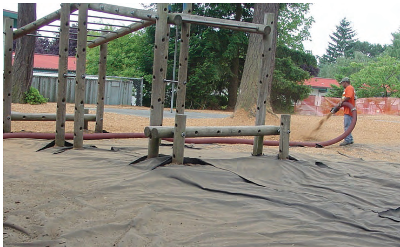
Images 2a and 2b. Covering soil with geotextile fabric and rubber matting or play chips
