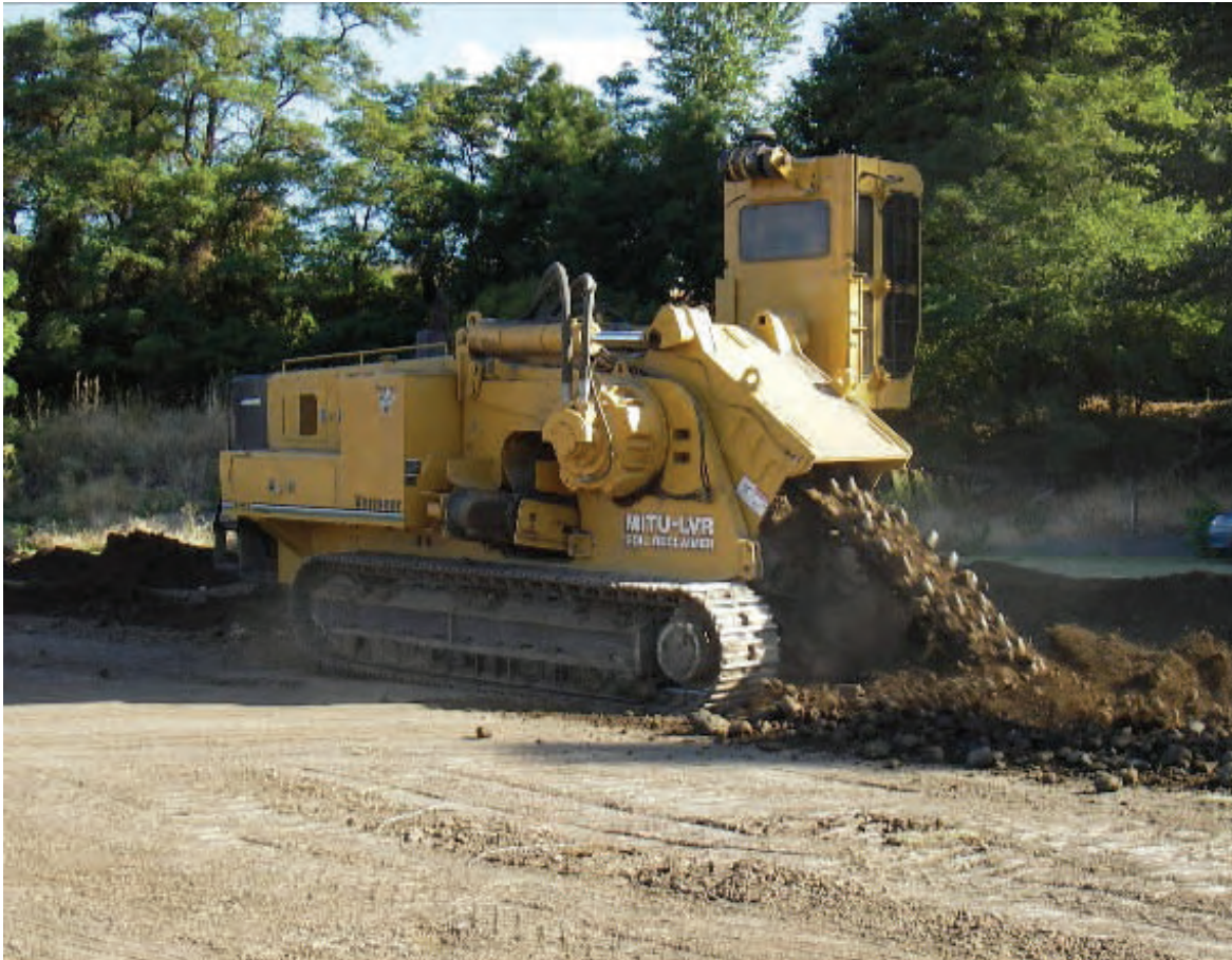
Image 12. Deep mixing at Naches Intermediate School, Yakima County
