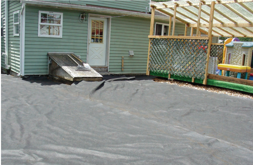
Image 10a. Geotextile barrier placed over soil
