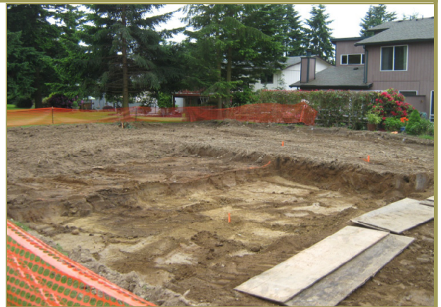
Excavating a new residential lot at Highland Hills
