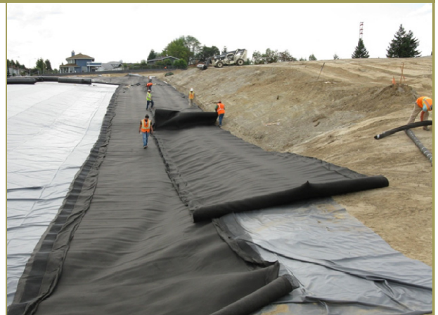
Laying a liner over the contaminated soil cell at StoneRidge
