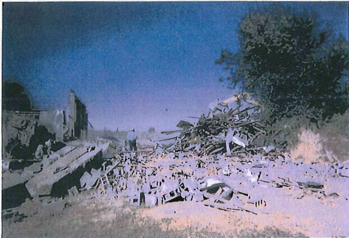
Photo 7 Demolition resumes (10/04/04) Photo taken by Breean Zimmerman
