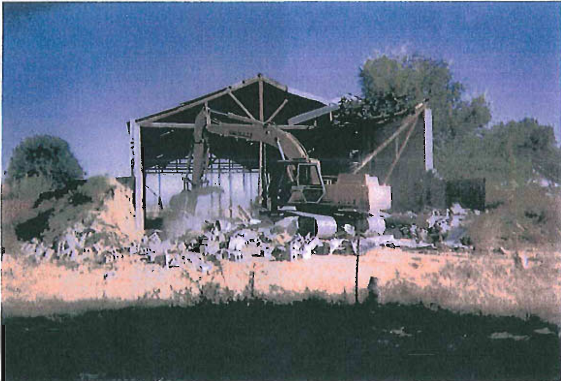
Photo 3 Demolition resumes (10/04/04) Photo taken by Breean Zimmerman
