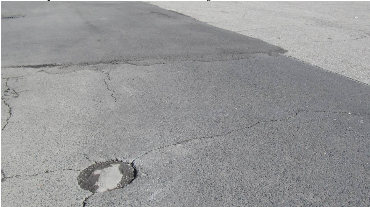
Photo 4: Asphalt Condition and Former Monitoring Well – from the northeast
