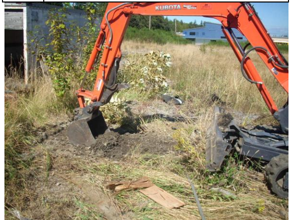
Photo #4: View of surficial petroleum stained soil being excavated at EX2-1.
