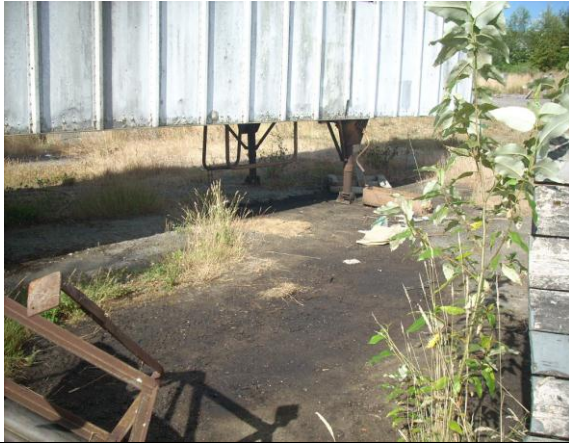
Photo #1: View of surficial petroleum stained soil near southeast corner of Site (see Figure 1, Site Plan , for aerial of site and sample location).
