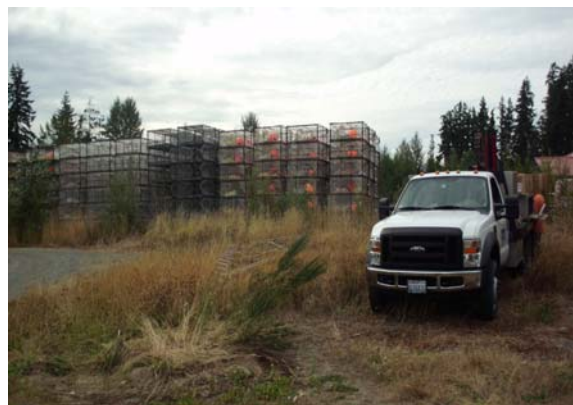
Photo #6: Direct push probe rig drilling at boring B-6 in Parcel C where documented hazardous materials were spilled on ground. View looking south.
