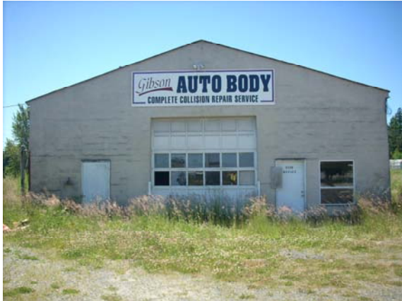
Photo #1: View looking southwest towards the main auto shop on former Gibson Auto Body (2328 Gibson Rd – at north end of Parcel A).
