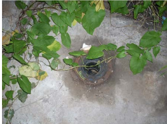
Photo #22: View looking at unknown drain in Parcel C garage. Note floor stains around drain.
