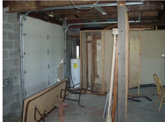
Photo #14: Representative view of condition and use of Parcel B house.
