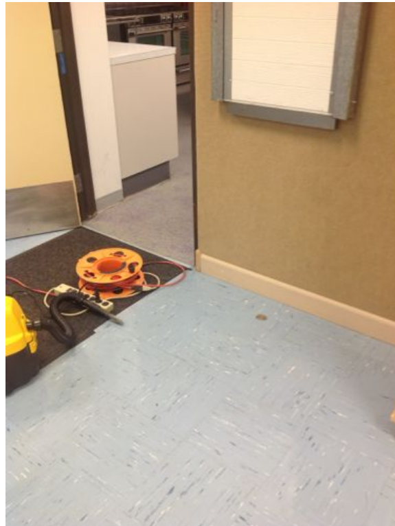
Photograph 20. Installed subslab sampling port at the Ridgefield Community Center, July 2013.
