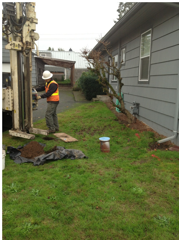
Photograph 12. Installing a soil gas sampling port outside the residence at 304 N 1st Avenue, November 2012.
