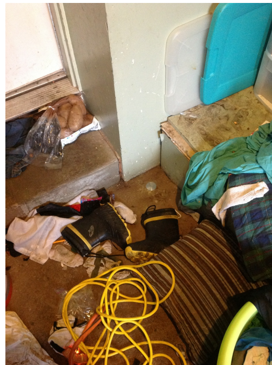
Photograph 16. Subslab port installed at 305 N Main Avenue, November 2012.
