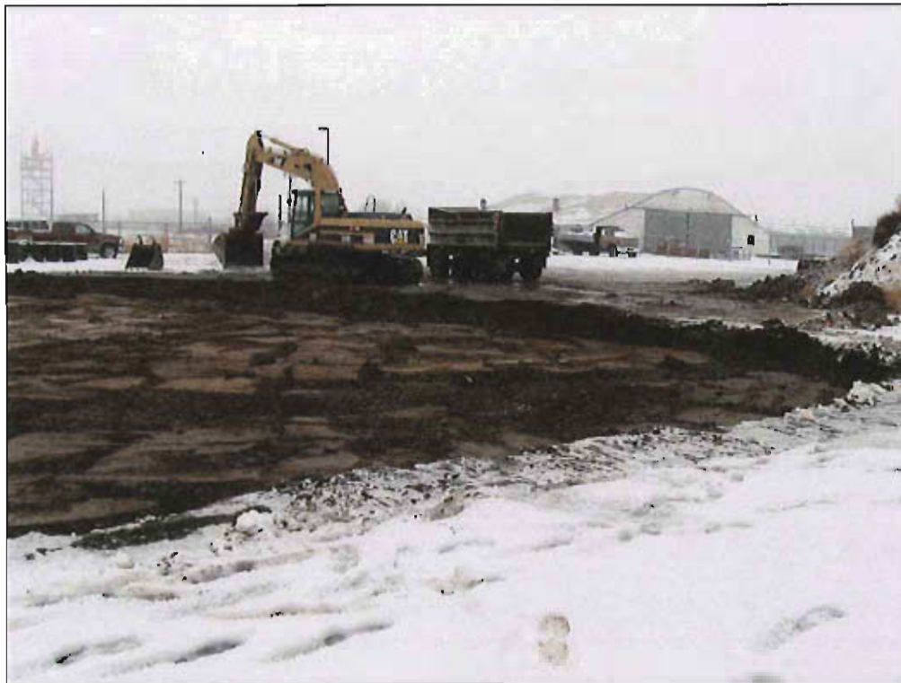
5. View of 2-ft excavation at north end of site (looking west from northeast edge). January 4, 2010.
