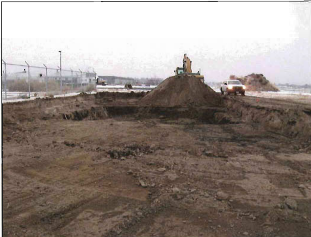
3. View of 3-ft and 6-ft excavations on west half of site (looking north). December 28, 2009.
