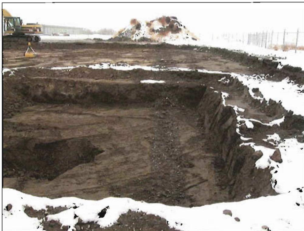
8. View of 6-ft excavation and gravel over stormwater drain line on east half of site (looking north). January 4, 2010.
