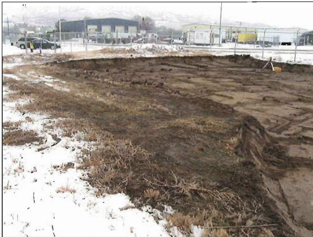
2. View of 2-ft excavation on south end of site (looking south-southwest from southeast edge of site). December 28, 2009.
