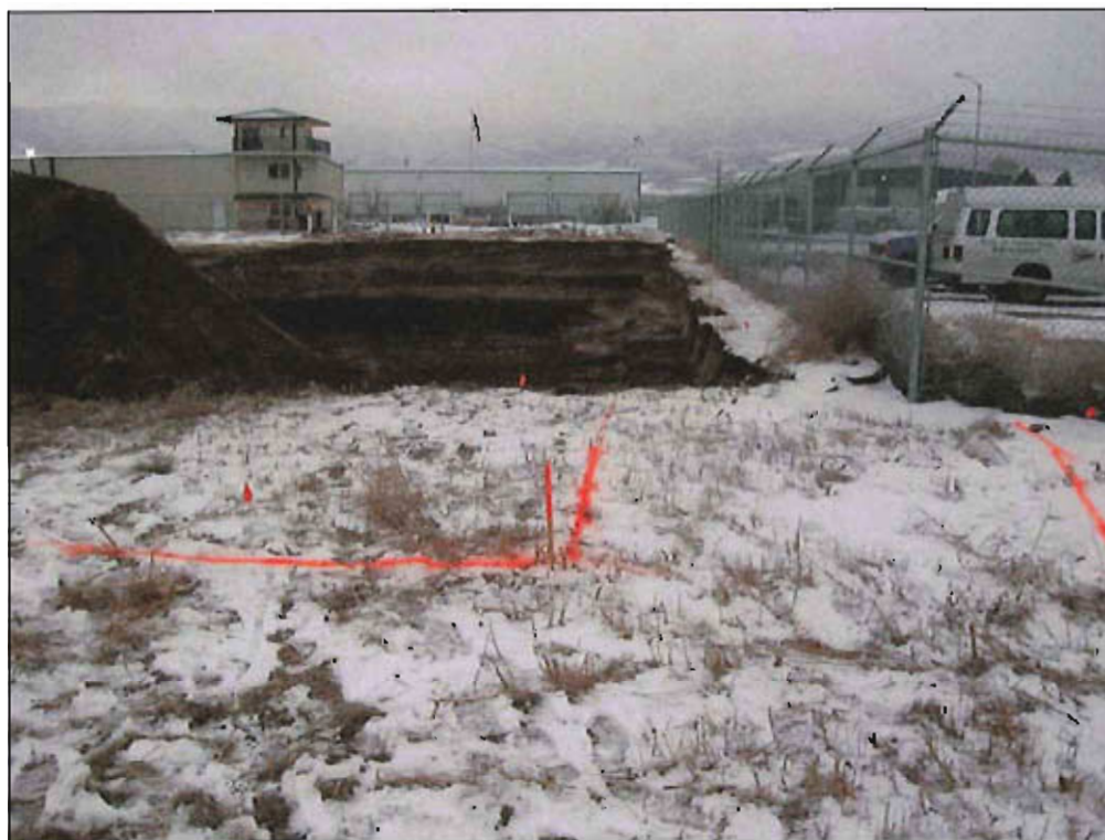
4. View of 3-ft and 6-ft excavations on west half of site (looking south). December 28, 2009.
