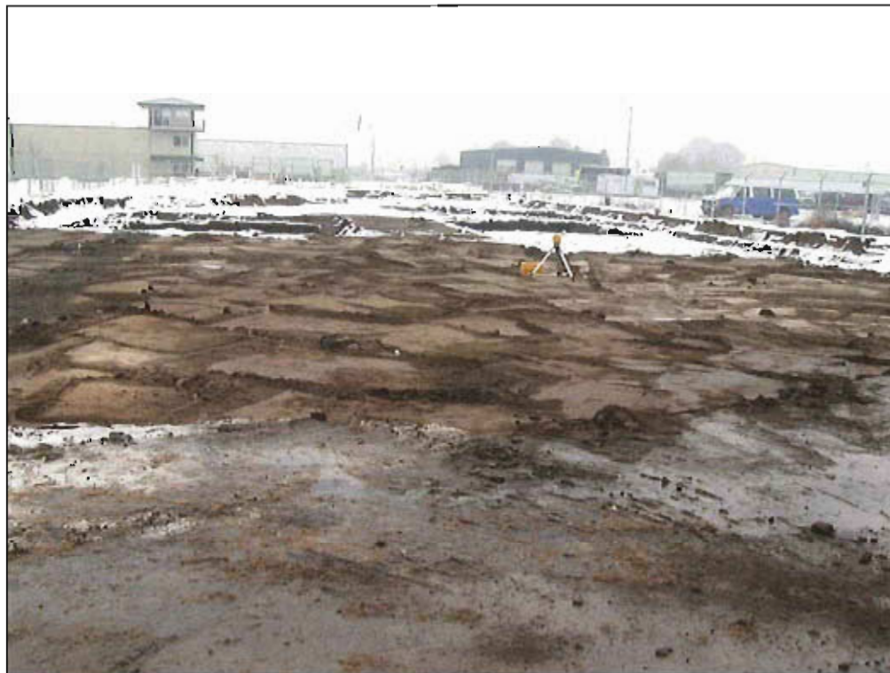
6. View from north end of excavation (looking south). January 4, 2010.
