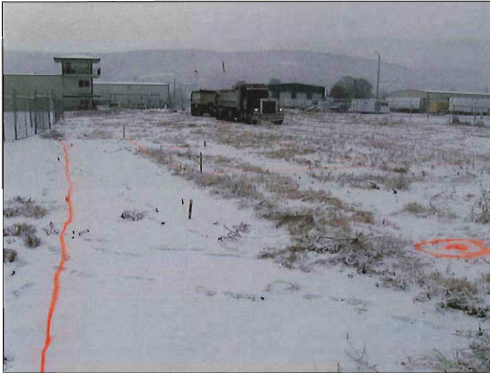
1. View of former washdown area prior to excavation (looking south from northeast corner of site). December 28, 2009.
