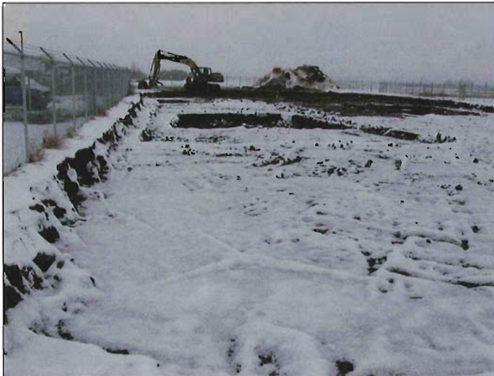
7. View from south end of excavation (looking north). January 4, 2010.
