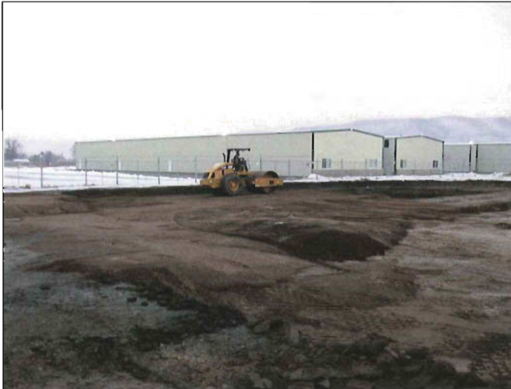
9. View of clean soil backfill on north end of excavation (looking east-southeast from northeast corner). January 11, 2010.
