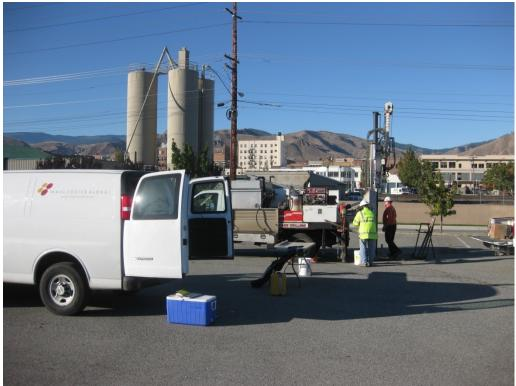
Photograph 9: View of the advancement of piezometer PZ1 in the west central portion of the Property. Photograph taken facing west.
