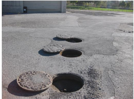
Photograph 17: Closer view of the oil/water separator located in the central portion of the Property.
