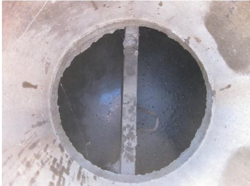
Photograph 14: View of the interior of the oil/water separator located in the east central portion of the Property.
