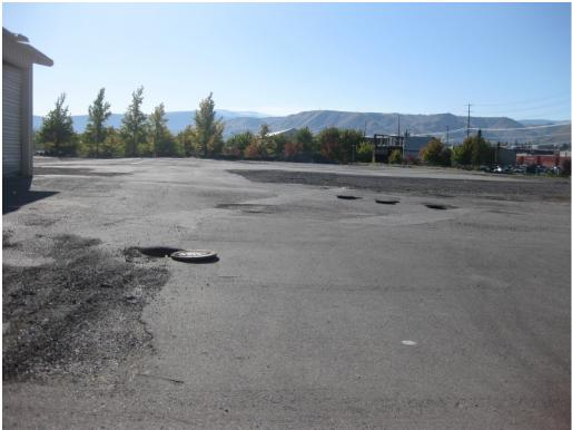
Photograph 15: View of a second oil/water separator (background) located in the central portion of the Property and a cleanout associated with the separators (foreground).
