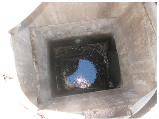
Photograph 18: View of the interior of the central oil/water separator at the Property.
