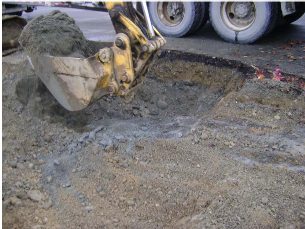
PHOTO 3: Excavation of top 2 to 3 feet, encounter and remove grey stained soil, 12/19/2011.
