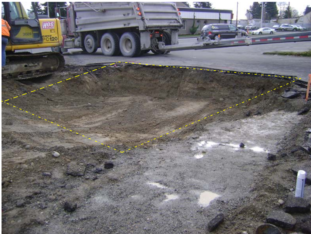
PHOTO 4: Final contaminated soil excavation limits on Lot' M' on 12/19/2011. Excavation limits are approximately 14-feet by 22-feet by 3 feet deep.
