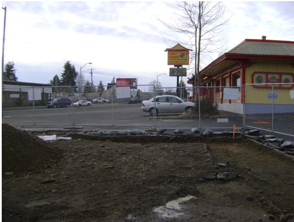
PHOTO 1: Graded surface lot and shallow curb footing trench, 12/13/2011, looking south.
