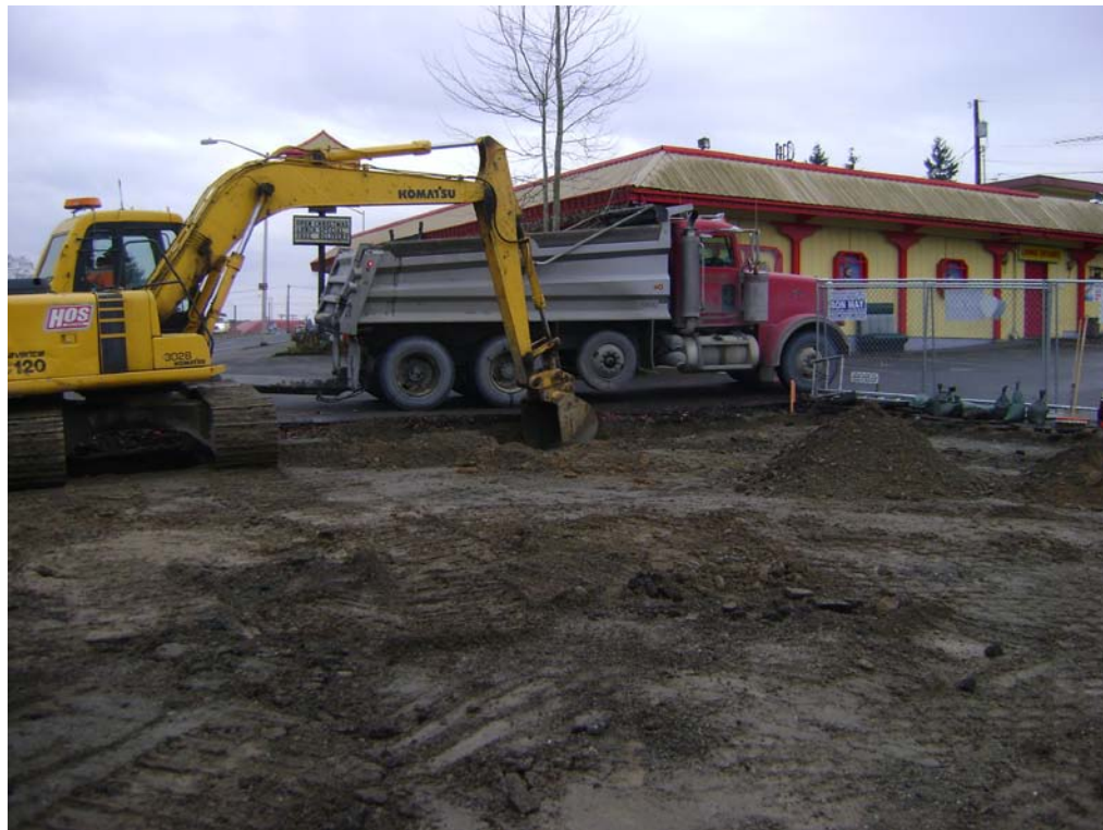
PHOTO 2: Petroleum contaminated soil excavation on 12/19/2011 on southwest portion of the Lot 'M' property.
