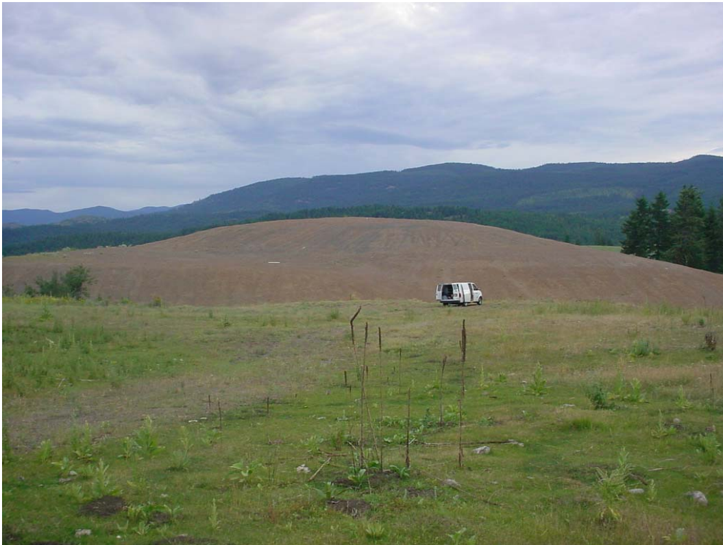
Photograph 1 - View of Waste Rock Pile 1 (WR-1).
