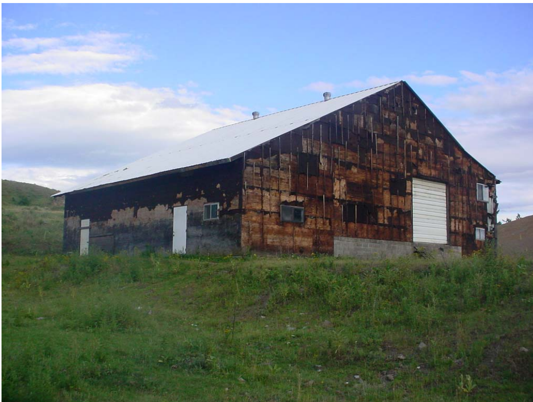
Photograph 6 - View of Building 1.
