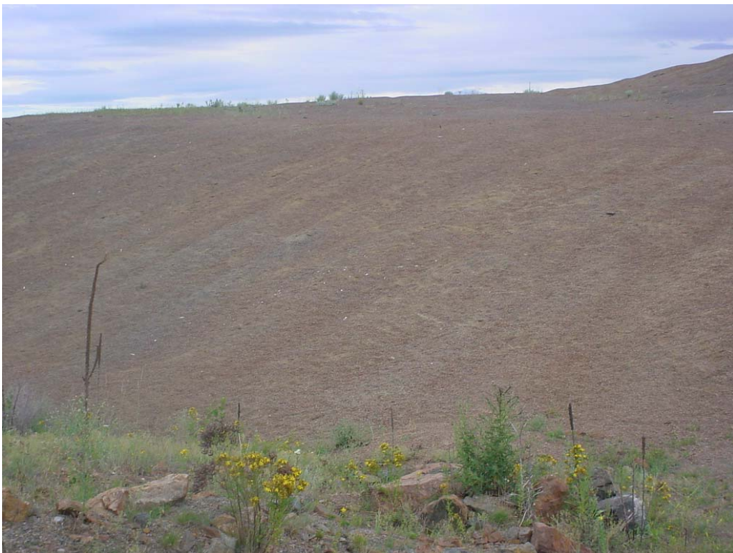
Photograph 2 - Example of drainage channels on WR-1.
