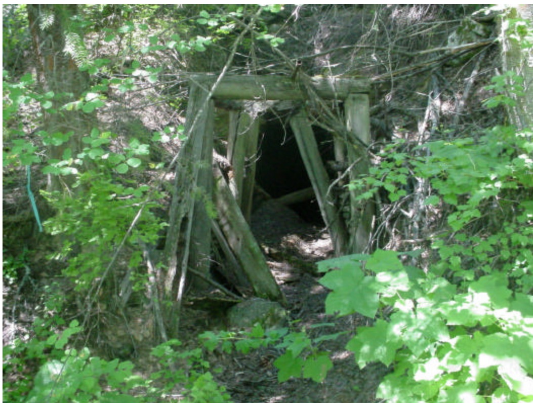
Photograph 3 - View of Adit 1 and support timbers
