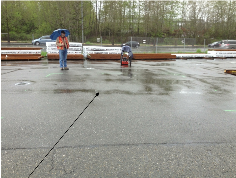
Possible UST pit
