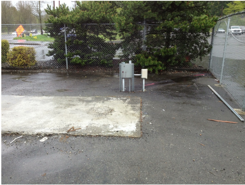
Electrical lines along perimeter fence
