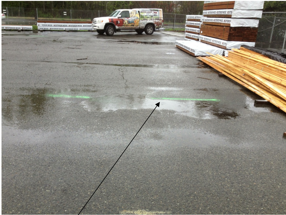
Unknown anomaly north of UST pit
