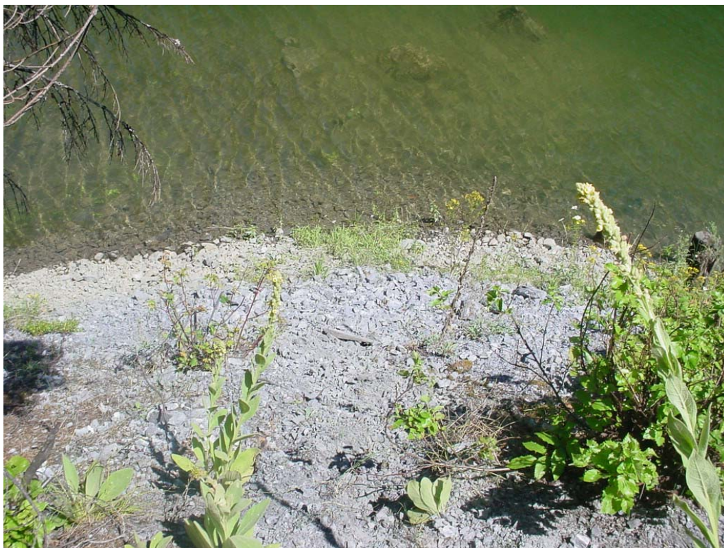
Photograph 2 - WR-1 showing Zone 3 material above and below the waterline.
