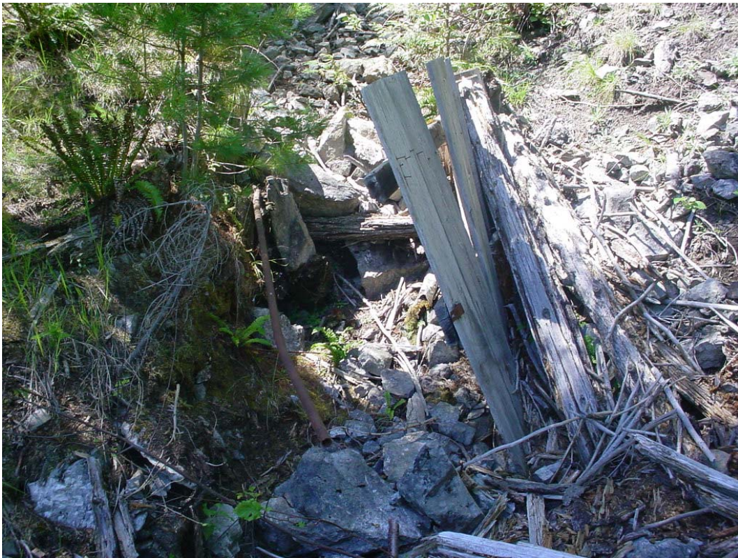
Photograph 3 - View of Adit-1.
