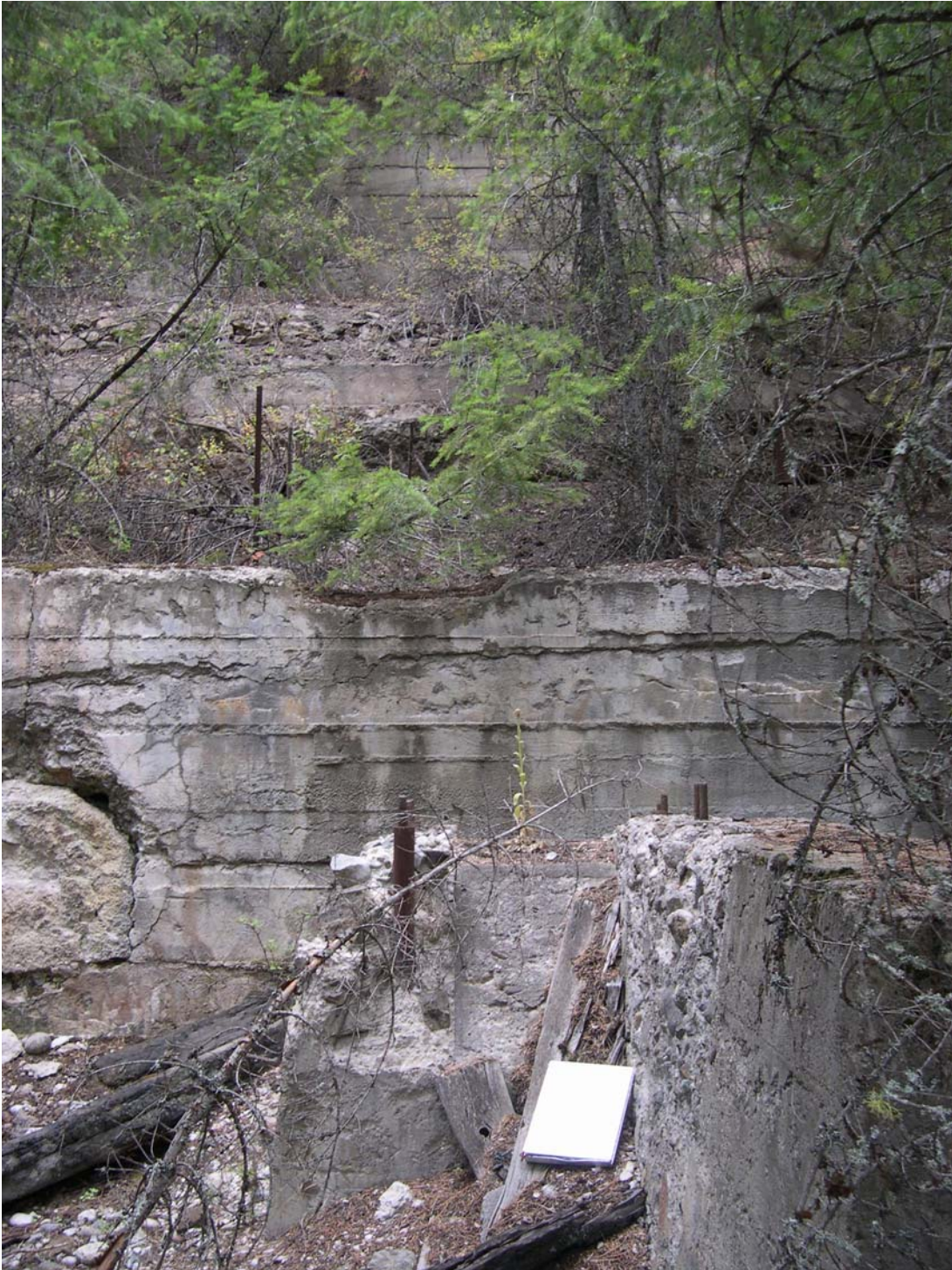
Photograph 2 - View of concrete foundations of former mill buildings.
