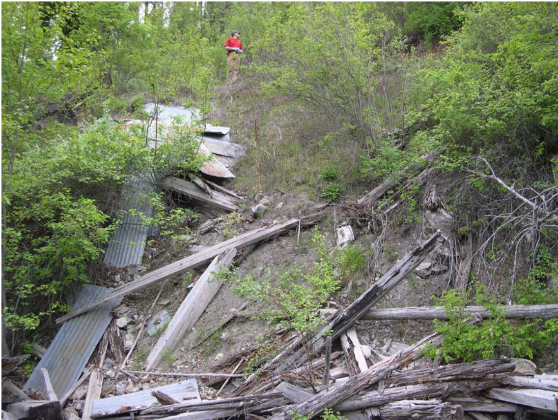
Photograph 5 - View of upper sections of WR-4 and DB-3.
