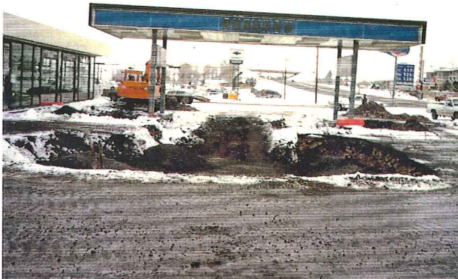
Site View Showing Tank Basin
