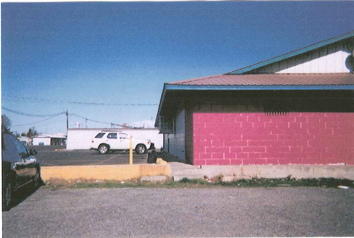
PHOTO 7: LOOKING NORTH ALONG THE EAST SIDE OF THE SUBJECT PROPERTY BUILDING
