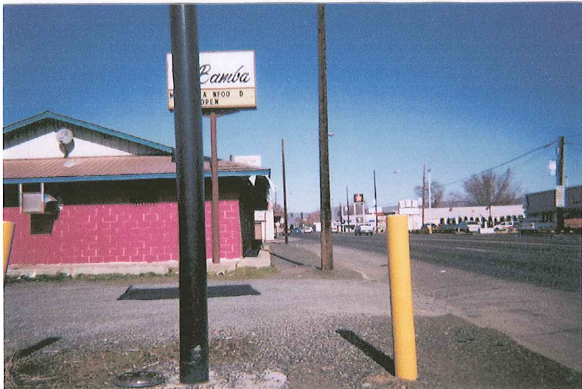
PHOTO 6: LOOKING NORTH ALONG THE EAST SIDE OF THE SUBJECT PROPERTY BUILDING
