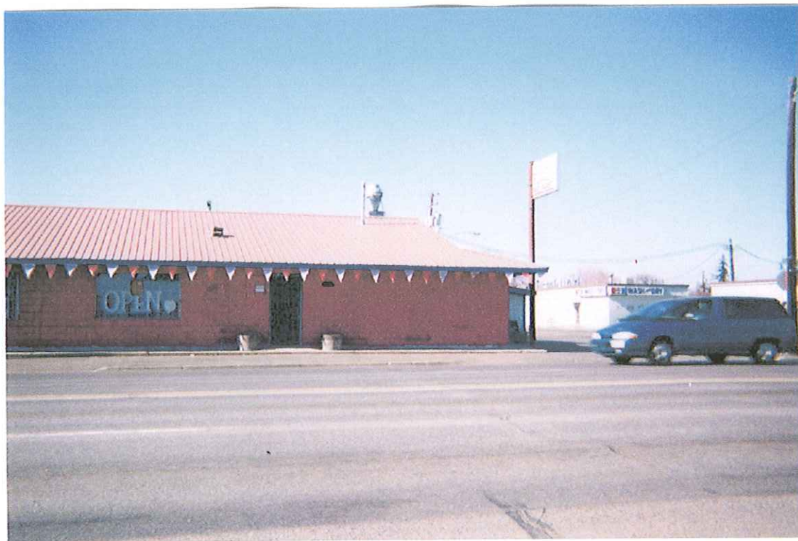
PHOTO 3: LOOKING WEST AT THE EAST SIDE OF THE SUBJECT PROPERTY BUILDING
