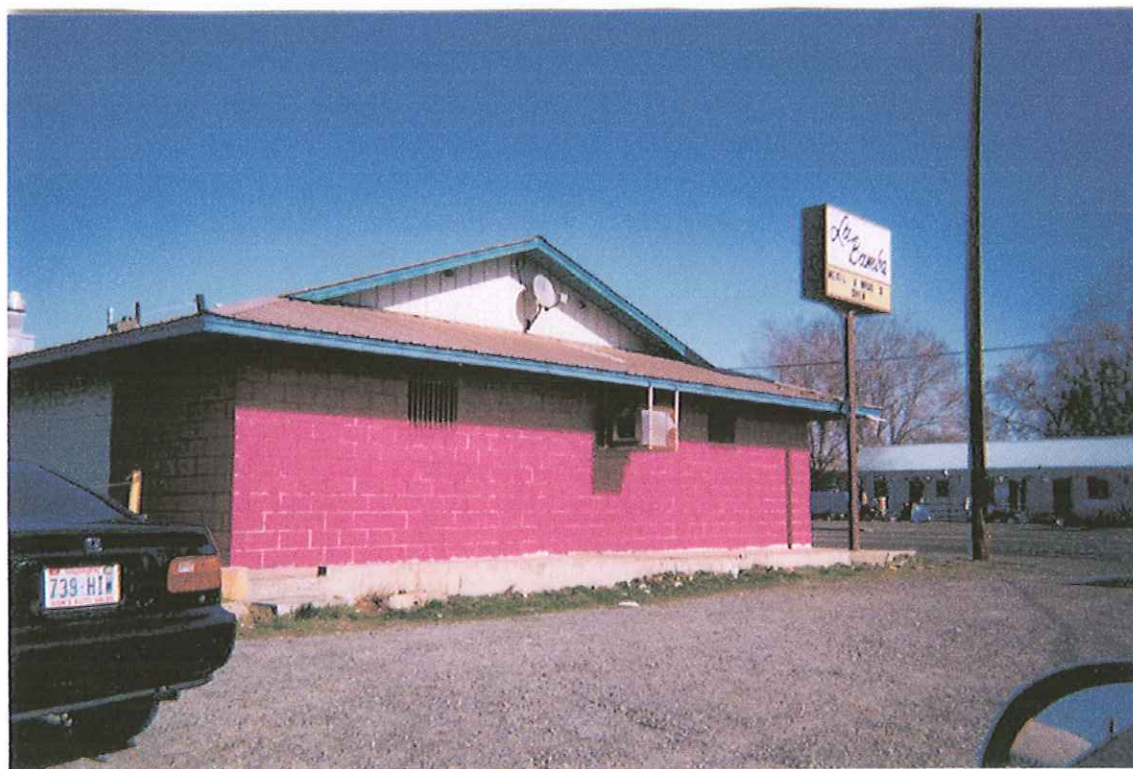
PHOTO 2: LOOKING NORTHEAST AT THE SOUTH SIDE OF THE SUBJECT PROPERTY BUILDING
