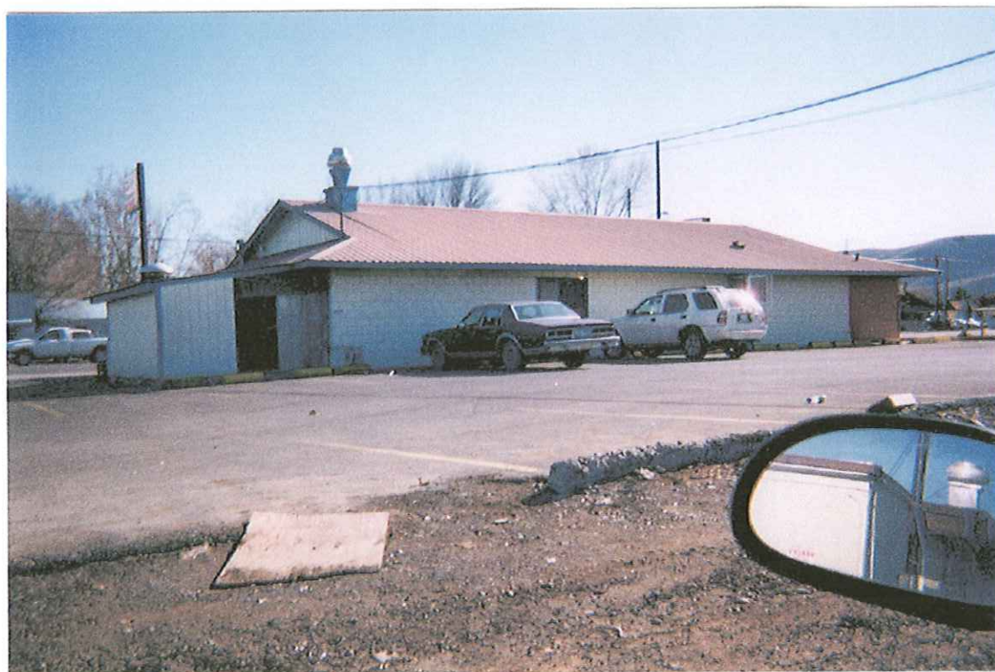
PHOTO 4: LOOKING SOUTHEAST ACROSS THE SUBJECT PROPERTY
