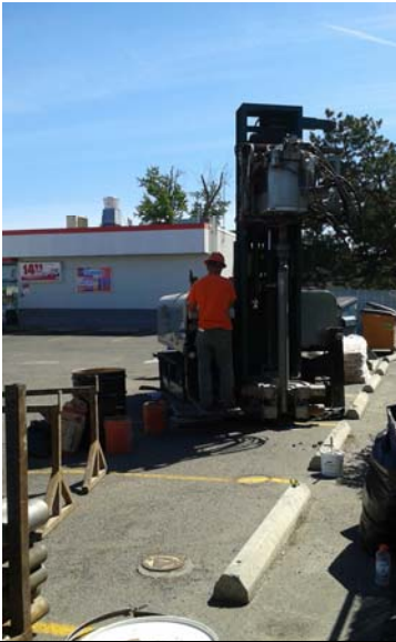
Photo #7: Location of Boring B-3 (Looking East)
