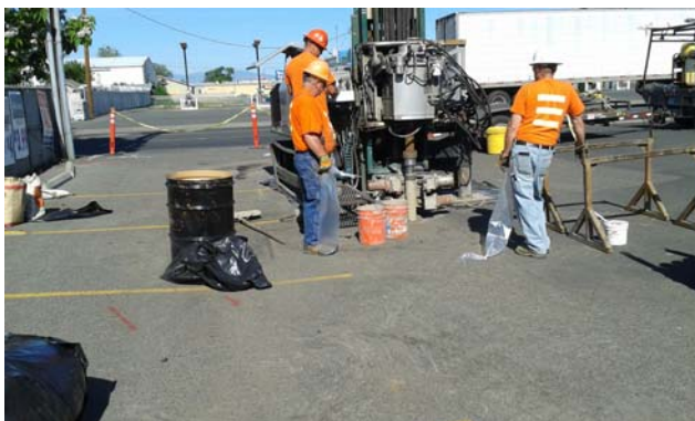
Photo #5: Location of Boring B-2 (Looking West)
