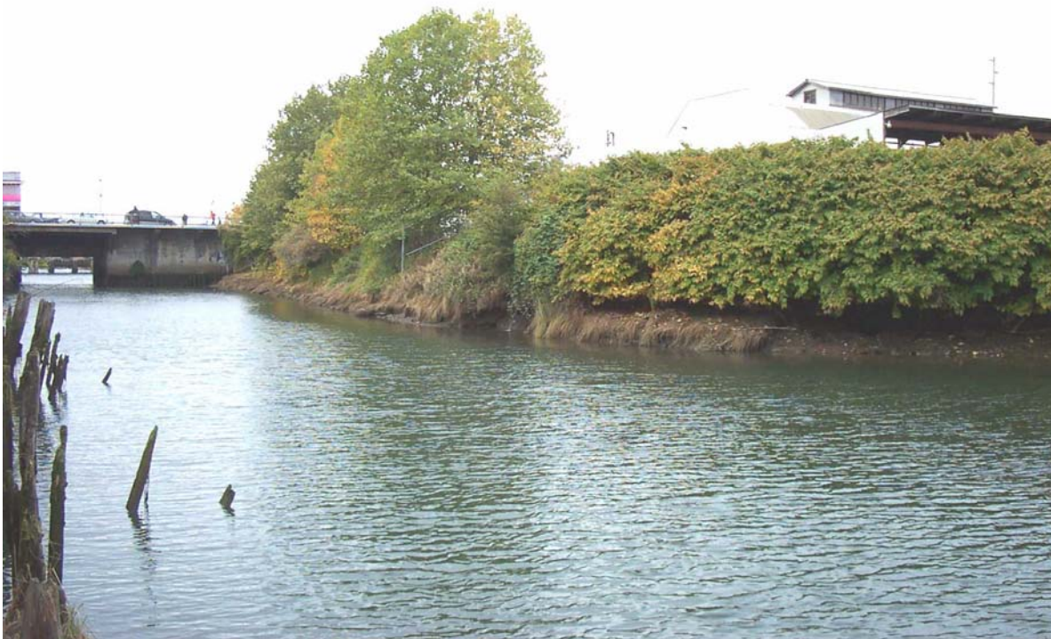
Photo 5-1. View of the existing shoreline slope and riparian vegetation along the north side of the Whatcom Creek Estuary.
