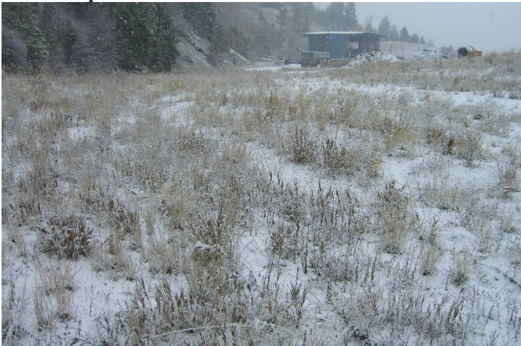
Photo 2: Landfill Cap – from the north
