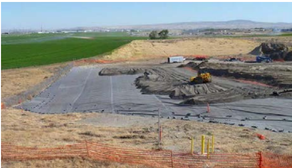
Construction of the New Zone B Cover
