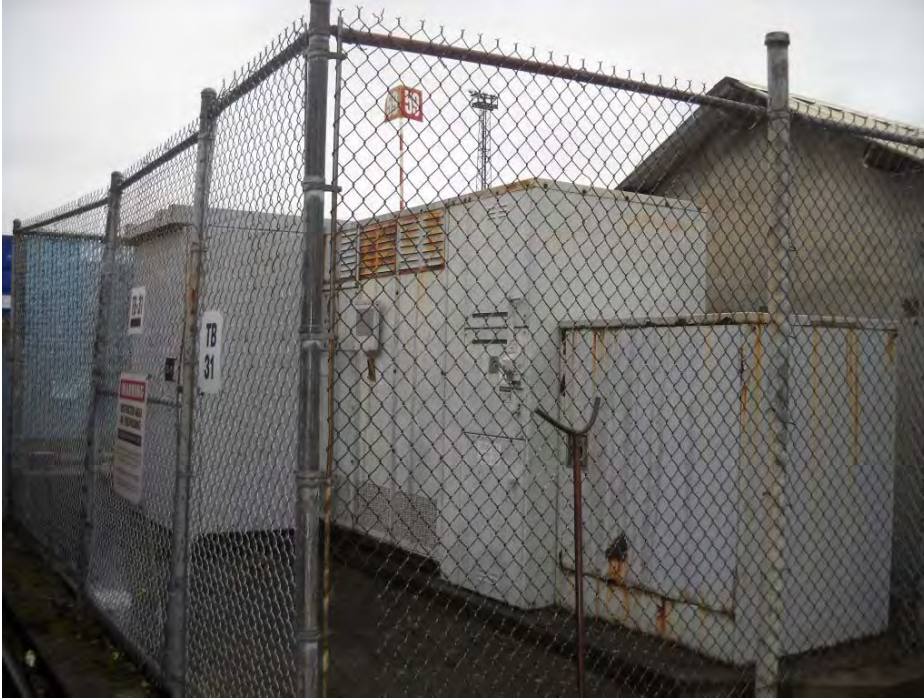
HSA No. 35. Electrical panels and wiring (M)
