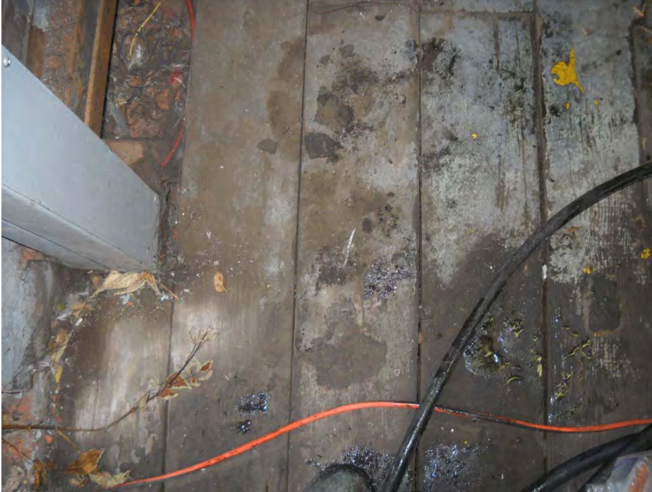
HSA No. 27. Brown residual floor sheeting (M)
