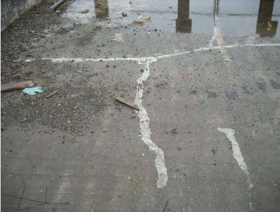
HSA No. 15. Light grey sealant (M)
