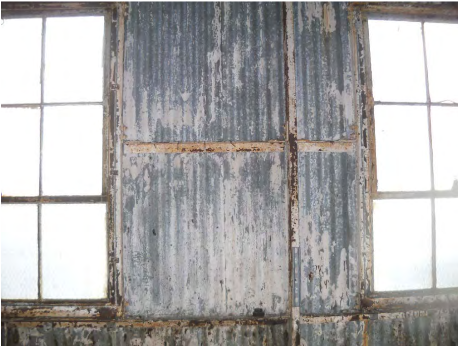
HSA No. 20. Silver paint and brittle material (M)
