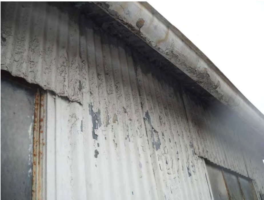
HSA No. 18. Off-white coating/sealant (M)
