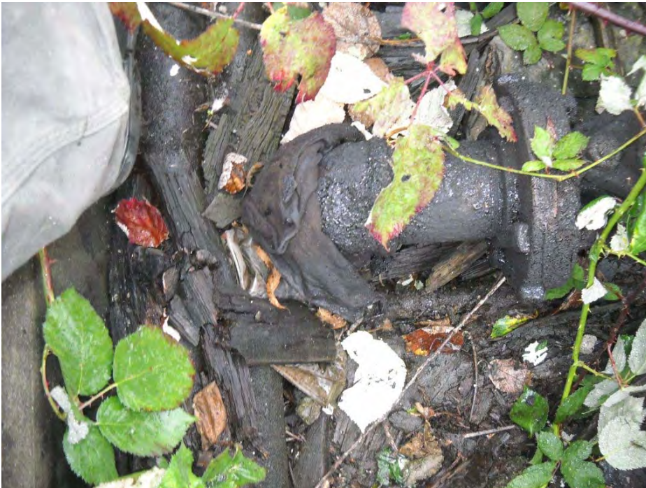
HSA No. 12. Black asphalt coating and canvas material (M)
