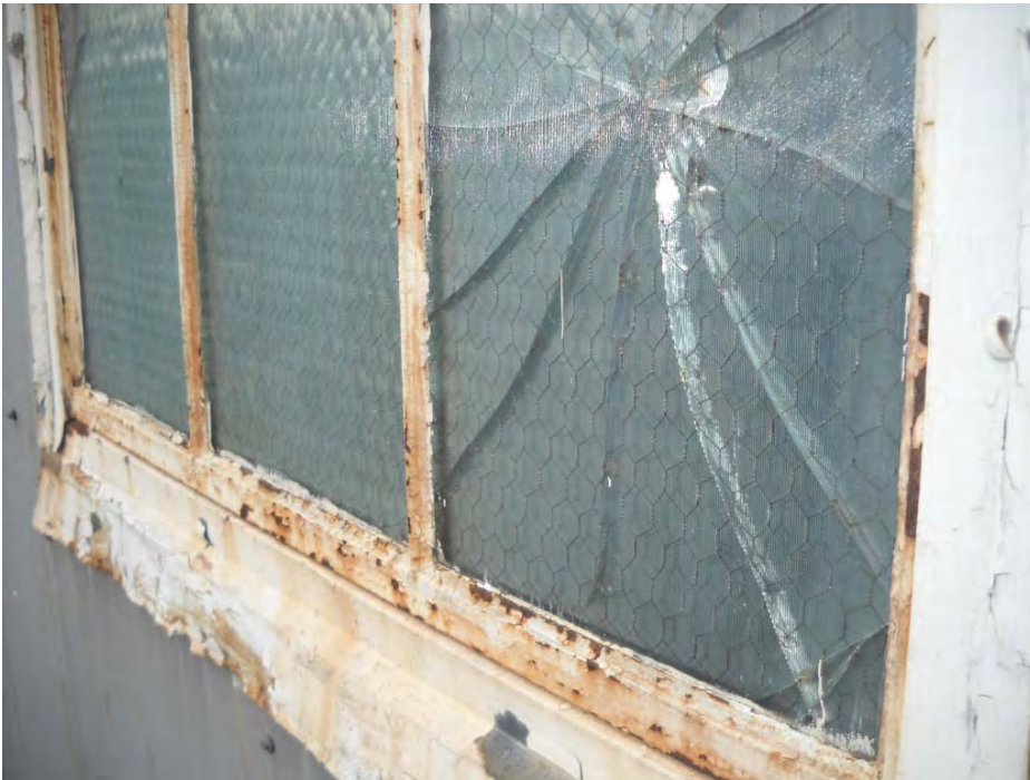
HSA No. 2. Grey exterior window glazing compound (M)
