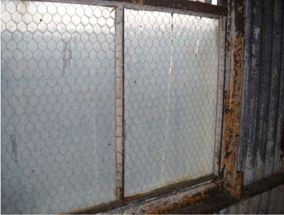
HSA No. 1. Grey interior window glazing compound (M)
