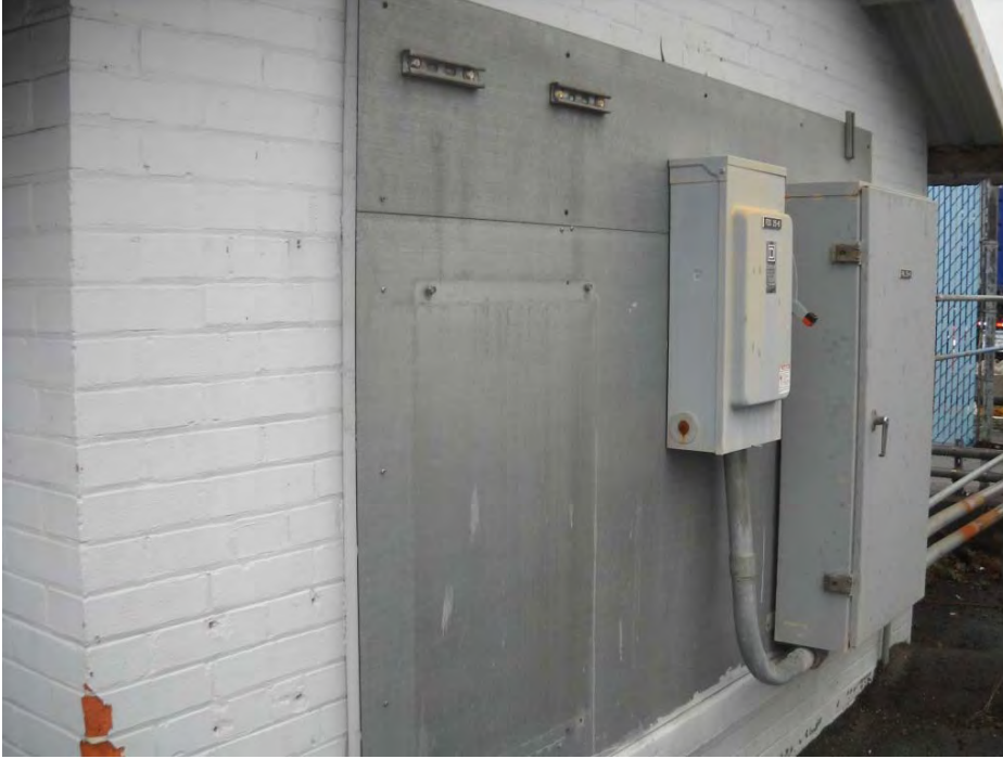
HSA No. 21. Grey exterior window glazing compound (behind metal panels) (M)
