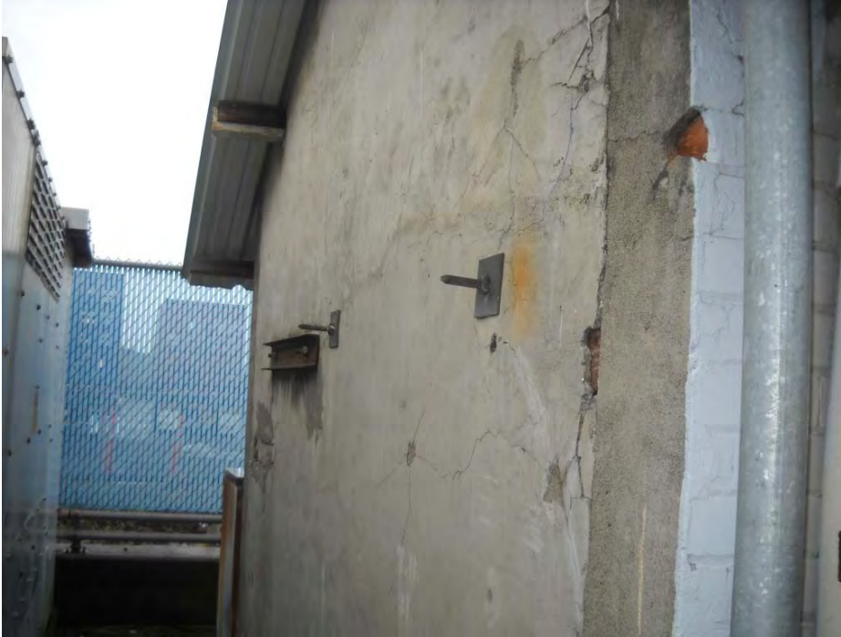
HSA No. 25. Grey stucco/plaster with metal lath (S)
