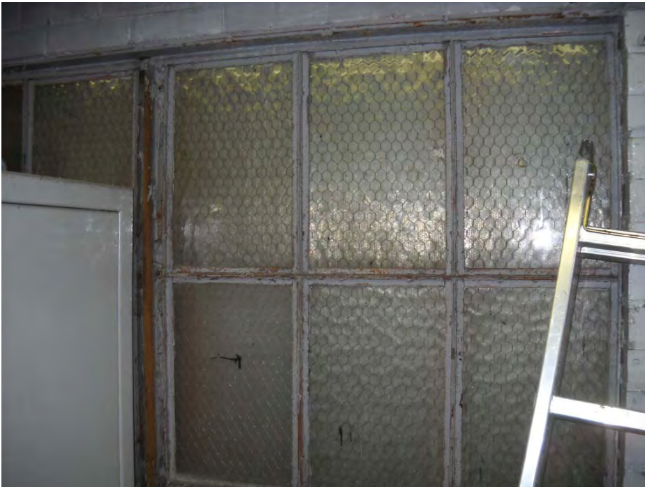
HSA No. 22. Grey interior window glazing compound (M)
