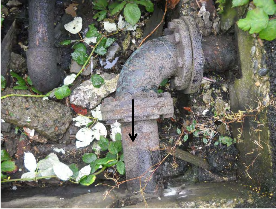
HSA No. 9. Black asphaltic coating (M)
