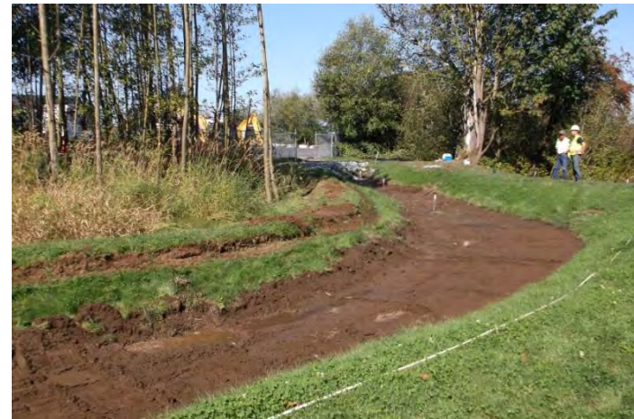
Photo 4. View of cleaned bioswale.
