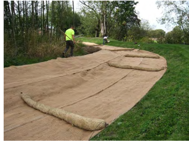
Photo 6. Jute matting and straw wattles were placed over the new topsoil.
