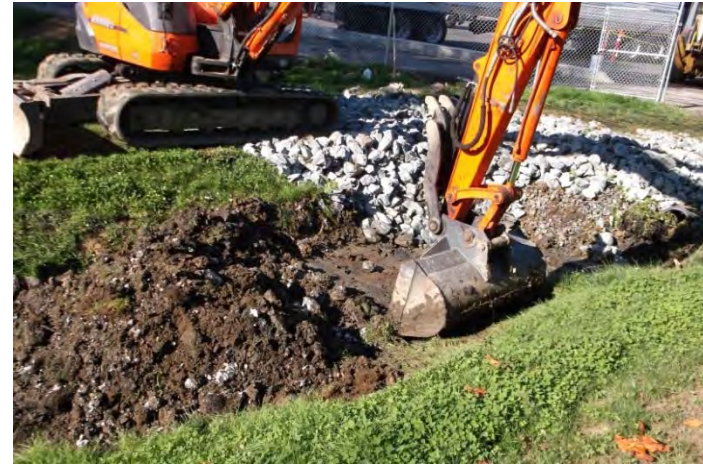
Photo 2. The stained soil was removed using an excavator.
