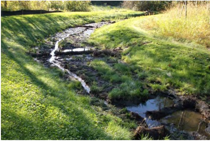
Photo 1. Stormwater bioswale prior to cleanup.
