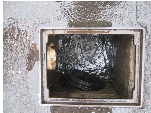
Photo 8. View of cleaned parking lot catch basin.
