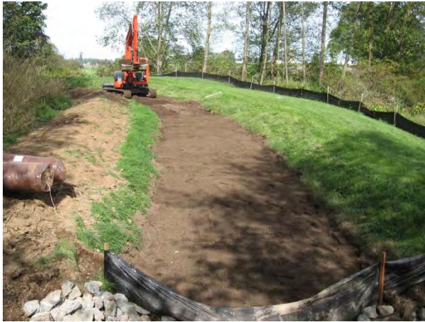
Photo 5. Topsoil was replaced in the clean bioswale.
