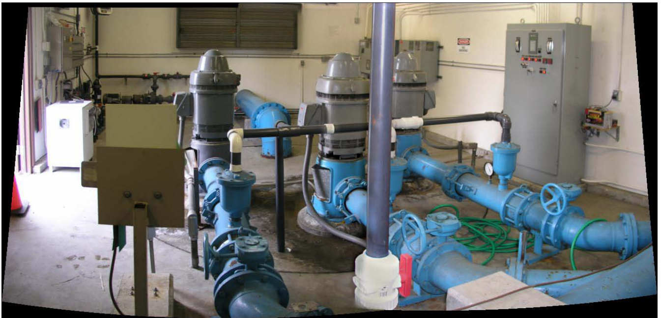
Inside treatment building with chlorination system
