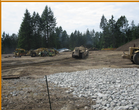
Creekside Village development site
