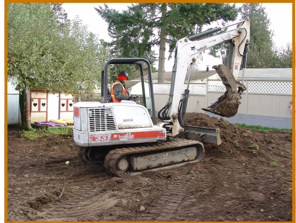
In most cases, we remove the top 12-18 inches of soil, then backfill and re-landscape the yard.
