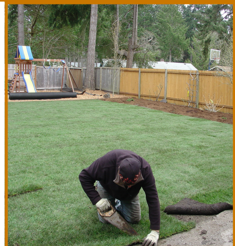
Cutting sod at the edge of a patio to finish re-landscaping a yard.
