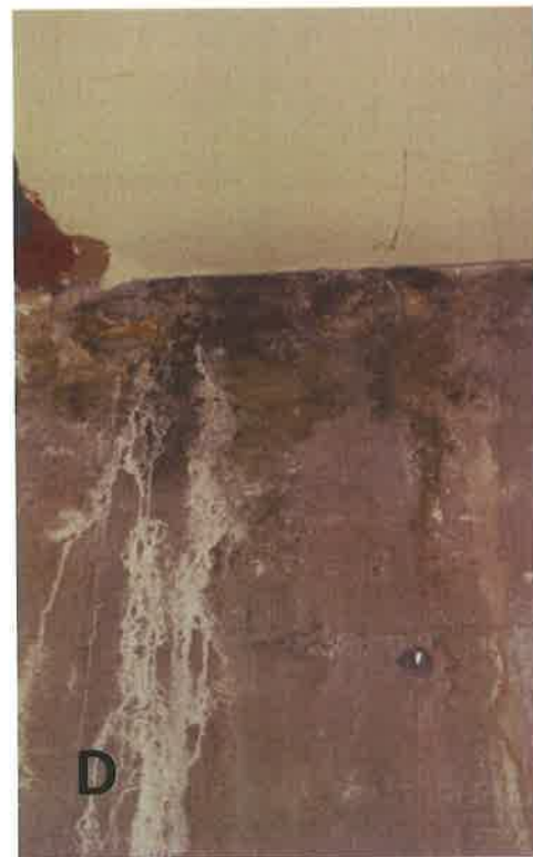
Figure 5. Site Photos. (A) Photo taken looking to west in alley behind building. Arrows show approximate locations where tanks were removed. (B) Close up of tank excavation in 1989. (C) Basement wall facing tank excavation area. (D) Evidence of seepage near the top of the wall in the cable vault.
