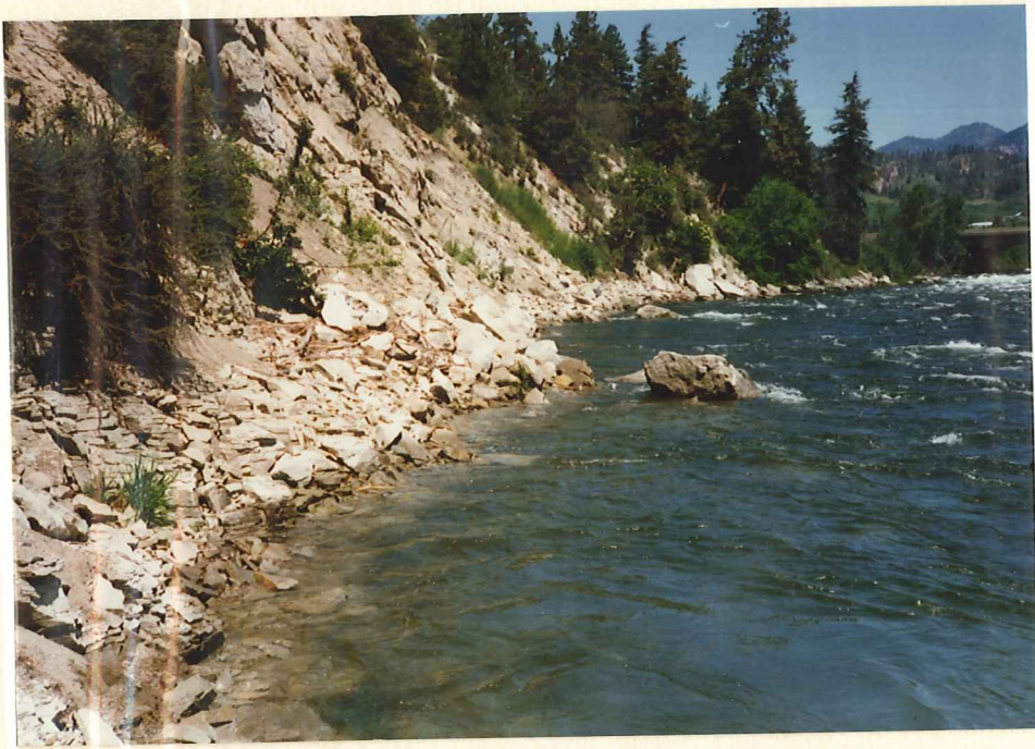
Photo 5 (above): View upriver from base of cliff during Phase I SI.
