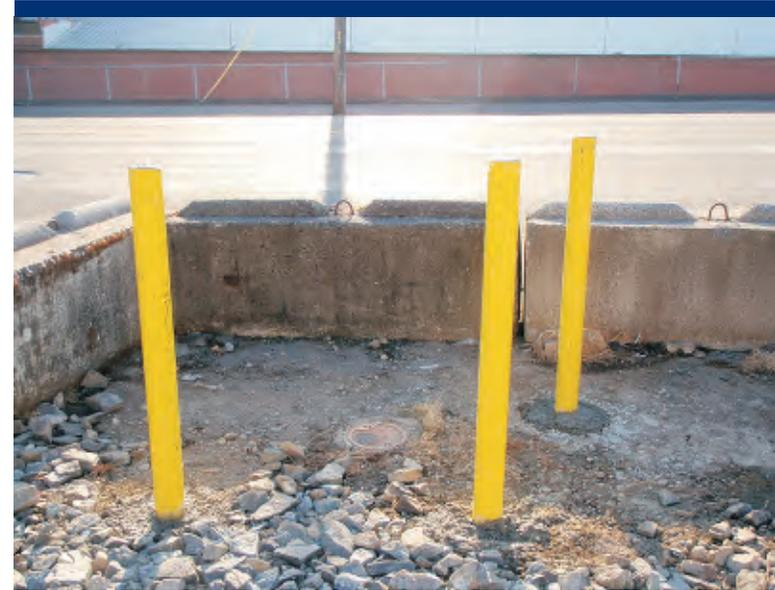
Photo 18 New bollards around MW1.
