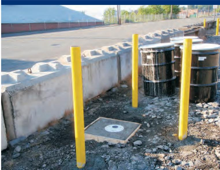
Photo 17 Completed monitoring well MW8.
