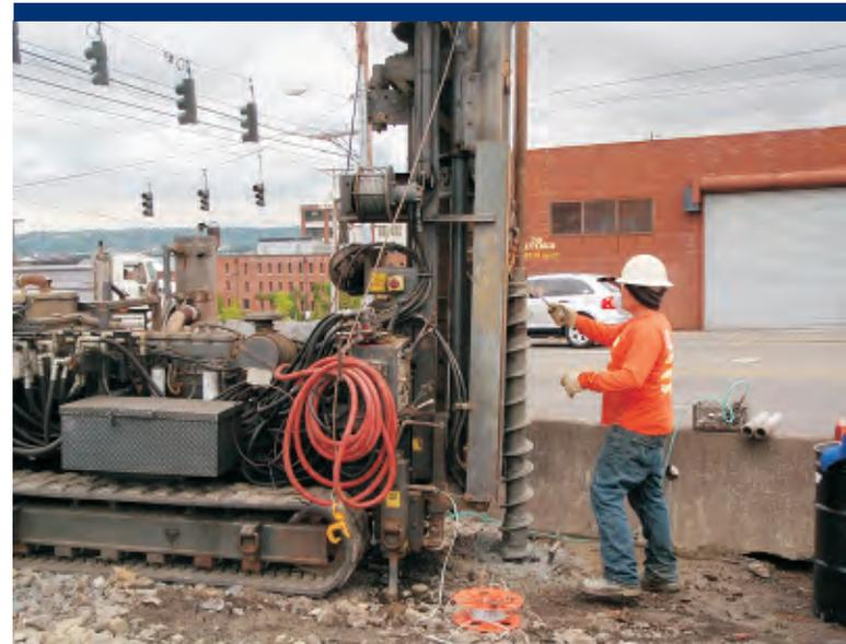
Photo 16 Installing monitoring well MW9.
