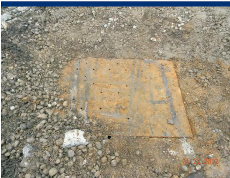
Photo 7 Metal lid of catch basin showing perforations.
