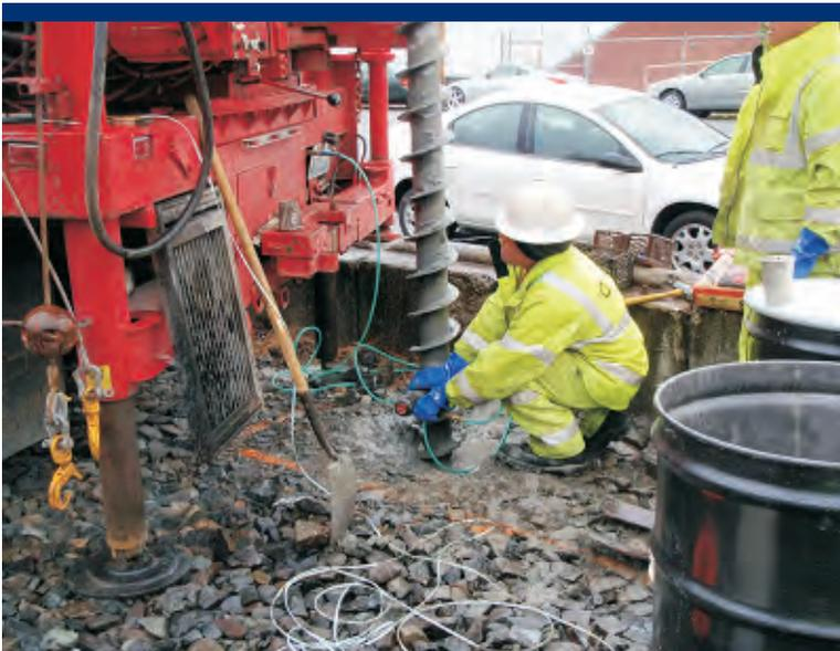
Photo 15 Installing monitoring well MW7.
