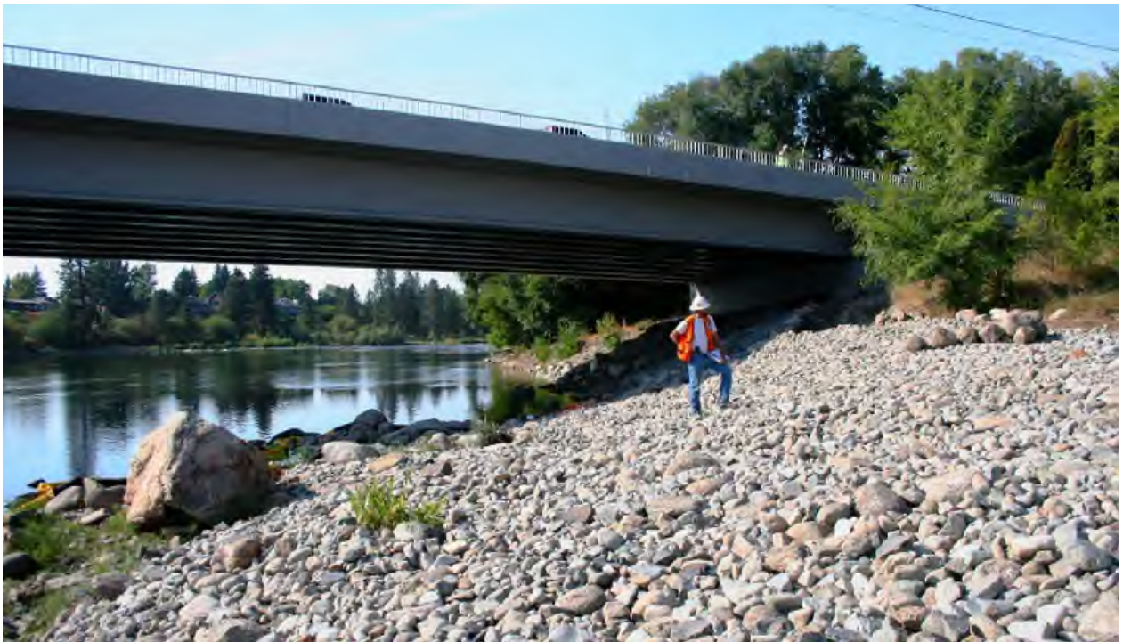
View of site facing west-northwest (downstream) during construction.
