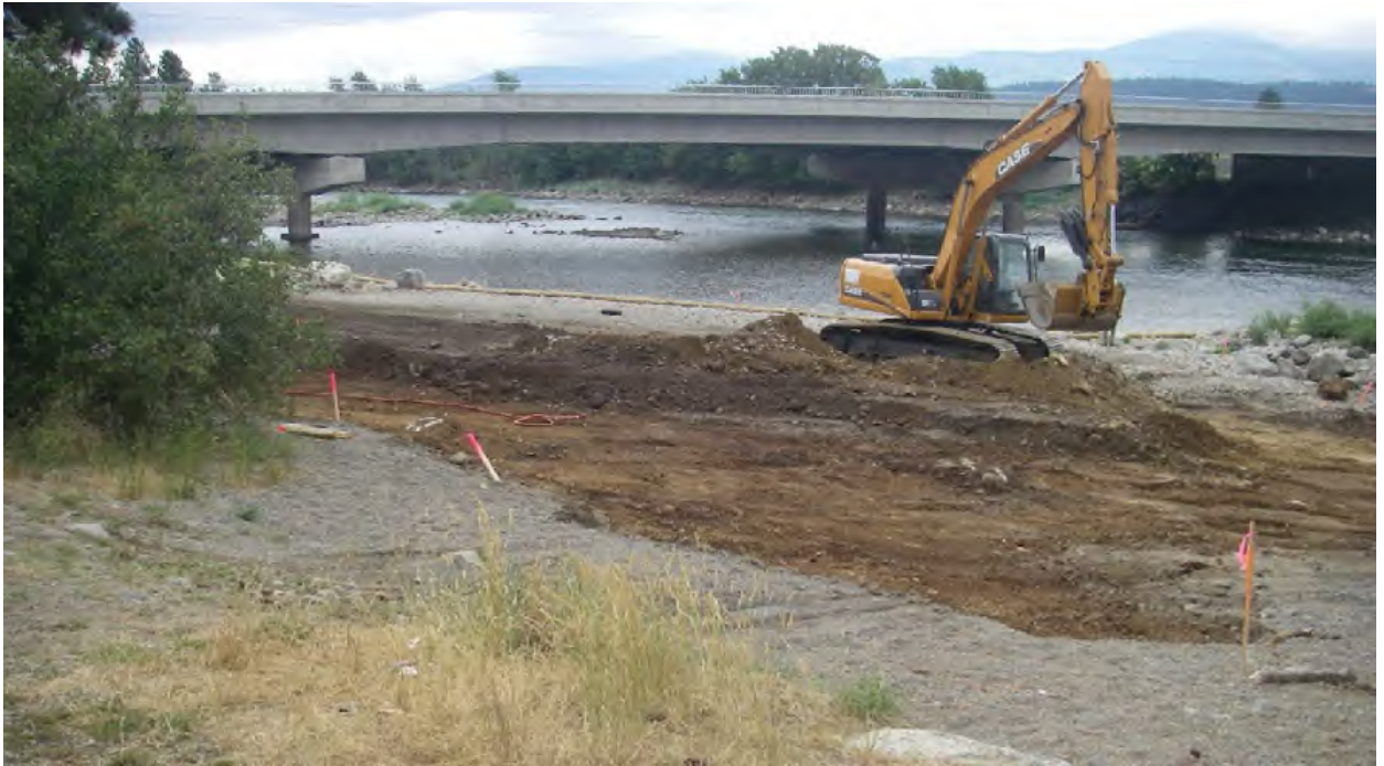
View from the site facing southeast during construction.
