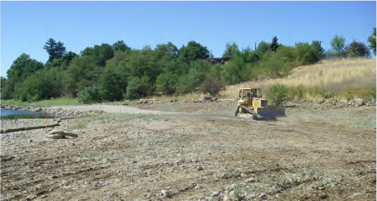
View of site facing west (upstream) during construction.
