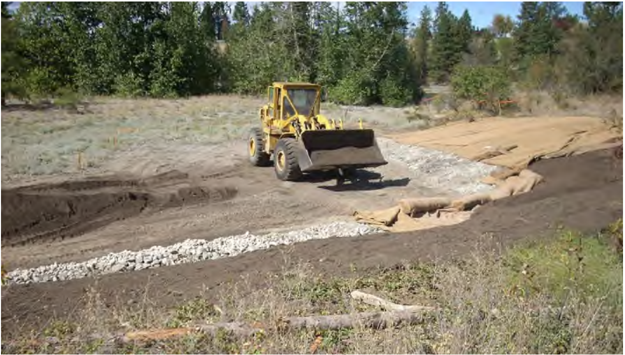
View from the site facing north during construction.
