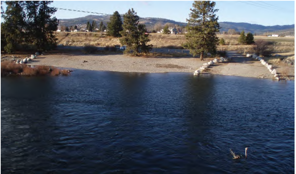
View of the site from the Harvard Road Bridge facing northwest post-construction.
