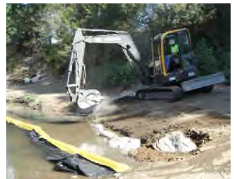
Below: Placing boulders along the southeast riverbank.
