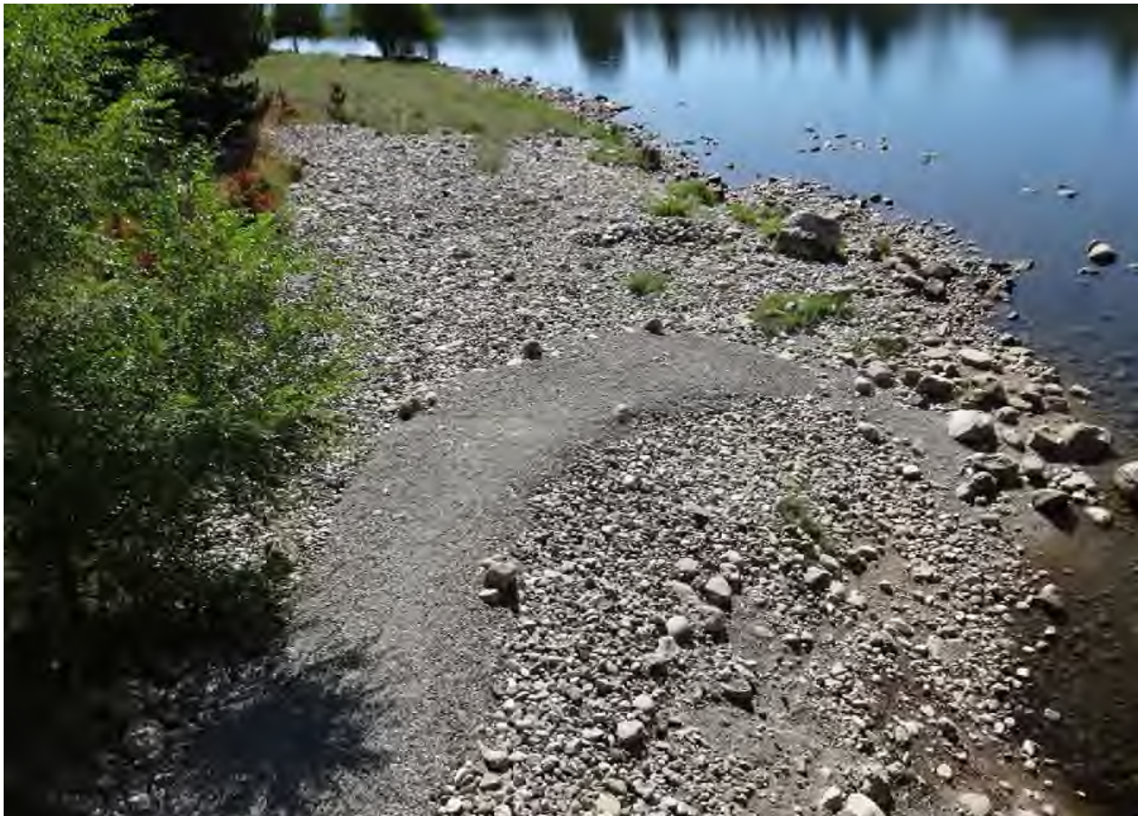
View of site from Barker Road North bridge facing east-southeast (upstream) post-construction.
