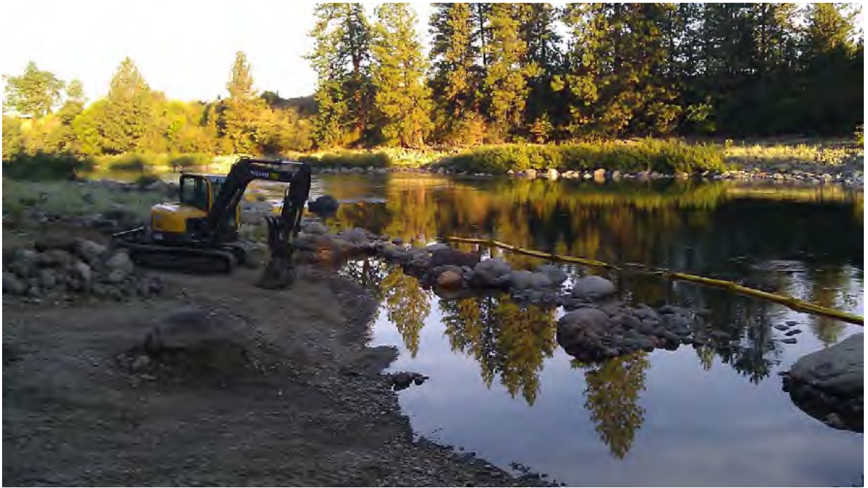
View of site facing west during construction.
