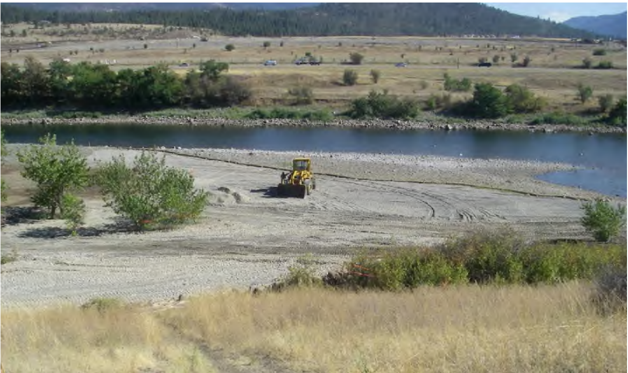
View of site facing south during construction.
