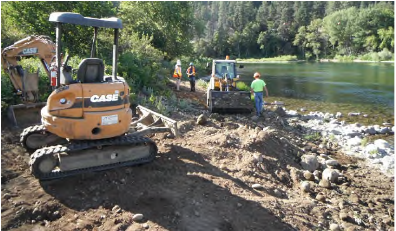
View of the site facing northwest (downstream) during construction.
