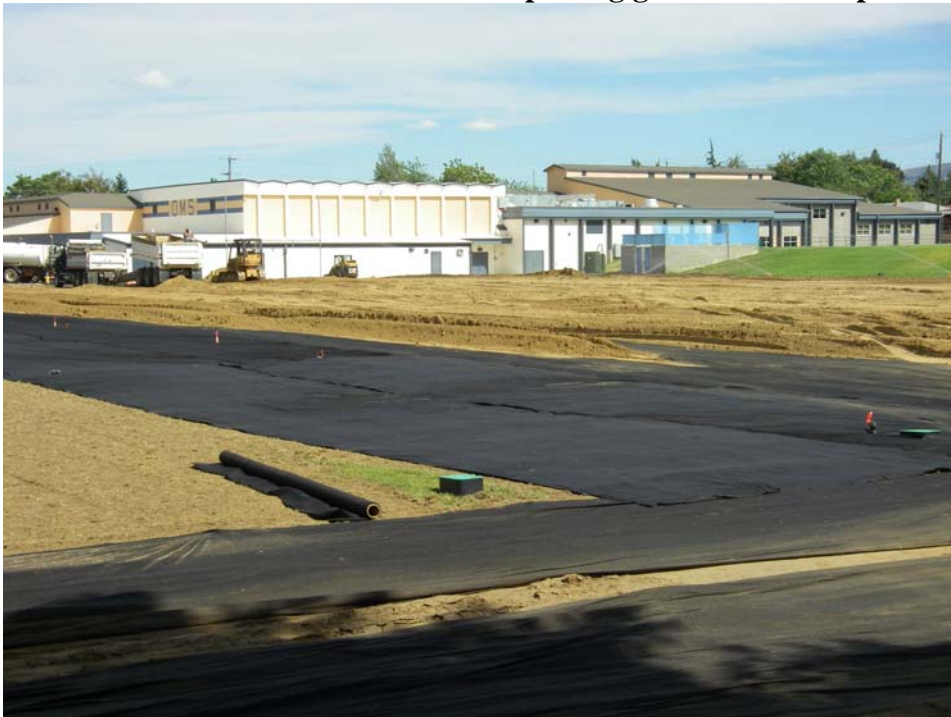
Photo D-2: Orchard Middle School placing geotextile and topsoil
