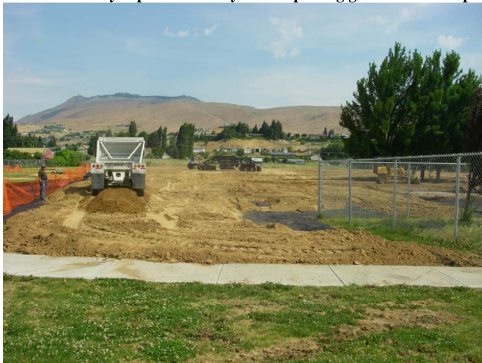
Photo D-2: Sunnyslope Elementary School placing geotextile and topsoil
