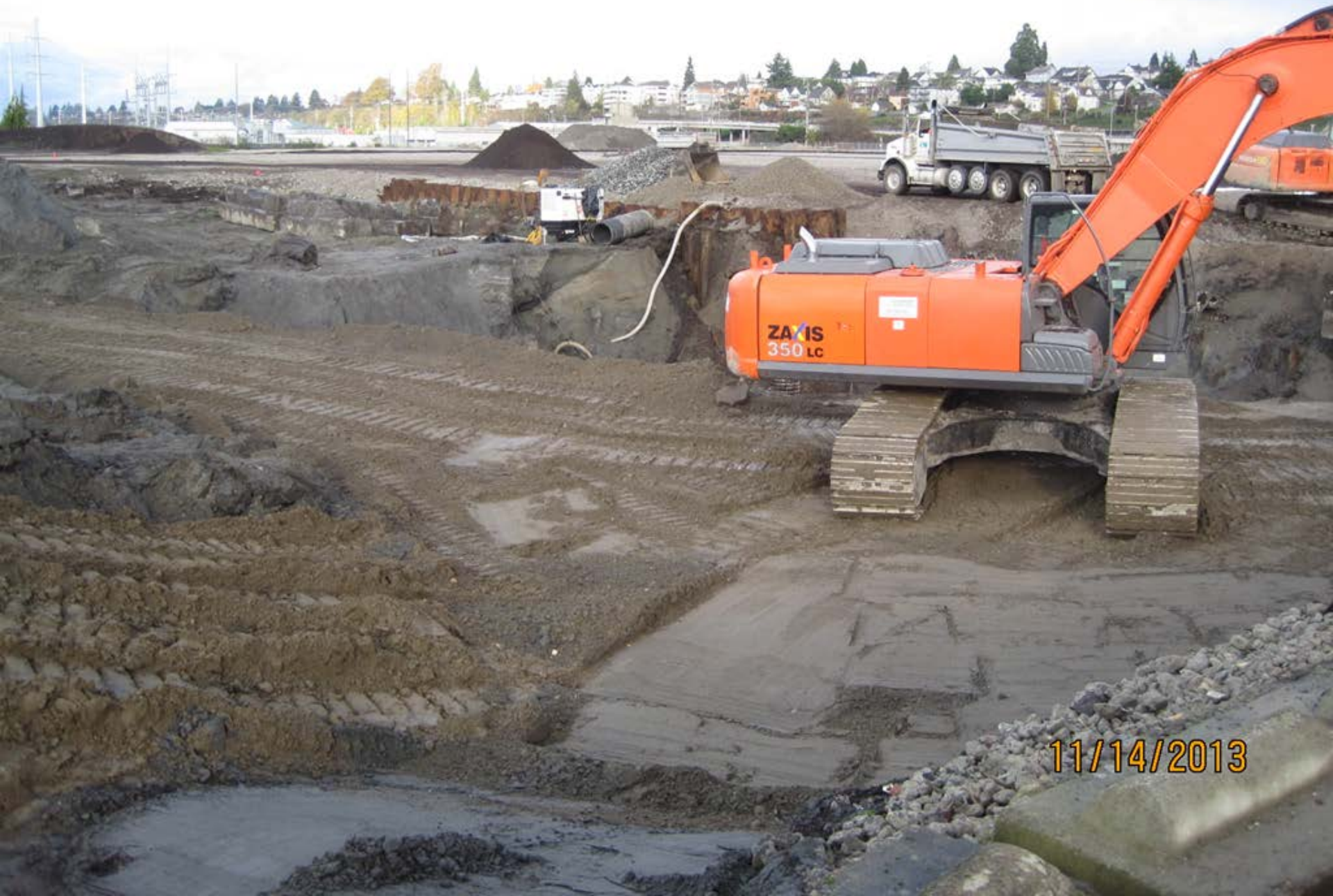
Excavation site at UST 70, view south east
