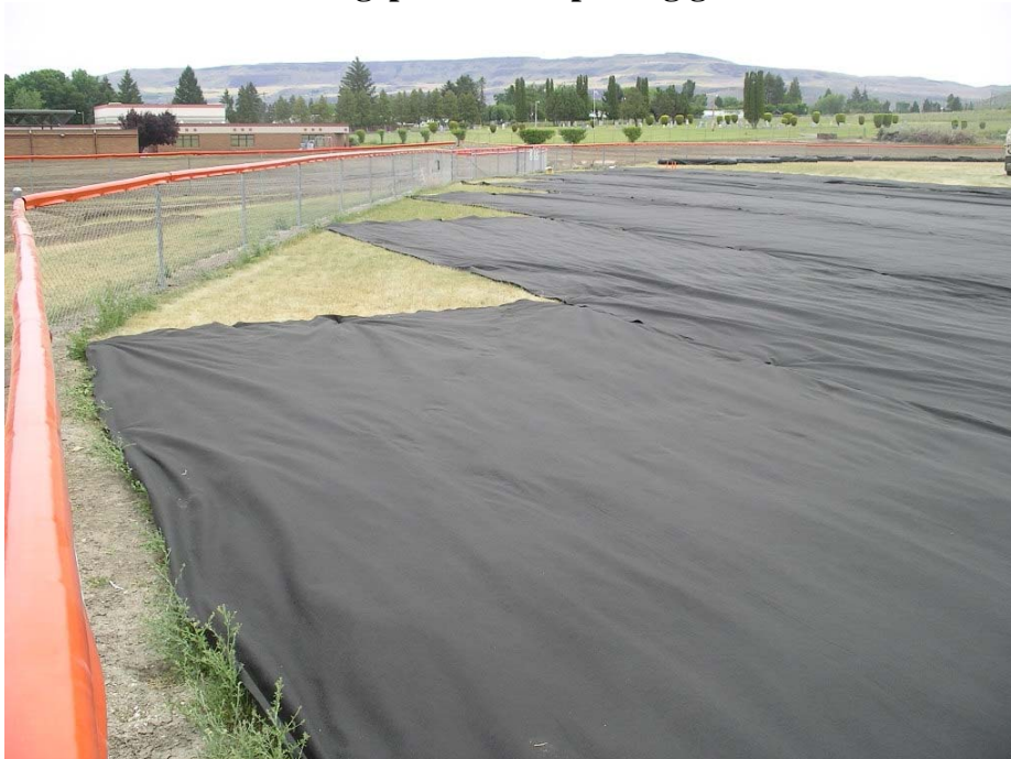
Photo D-2: Bridgeport School placing geotextile liner
