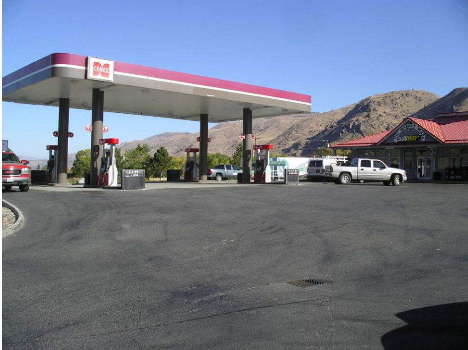
Photo 1: Front of Facility - from the southeast
