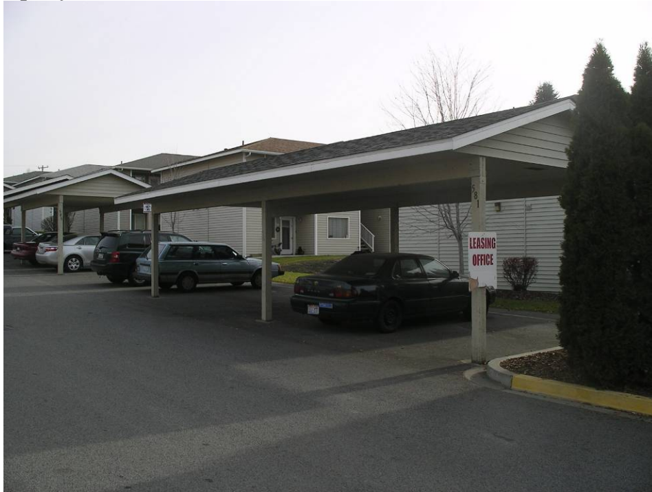
Photo 1: Property Entrance - from the northwest
