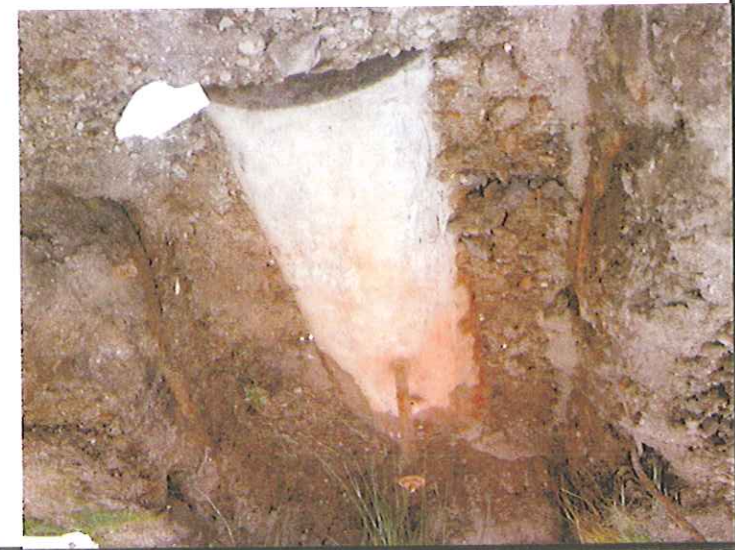
Unearthed 550-gallon gasoline UST, awaiting Fire Marshal inspection prior to removal.
