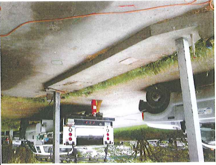
Former pump island area.
