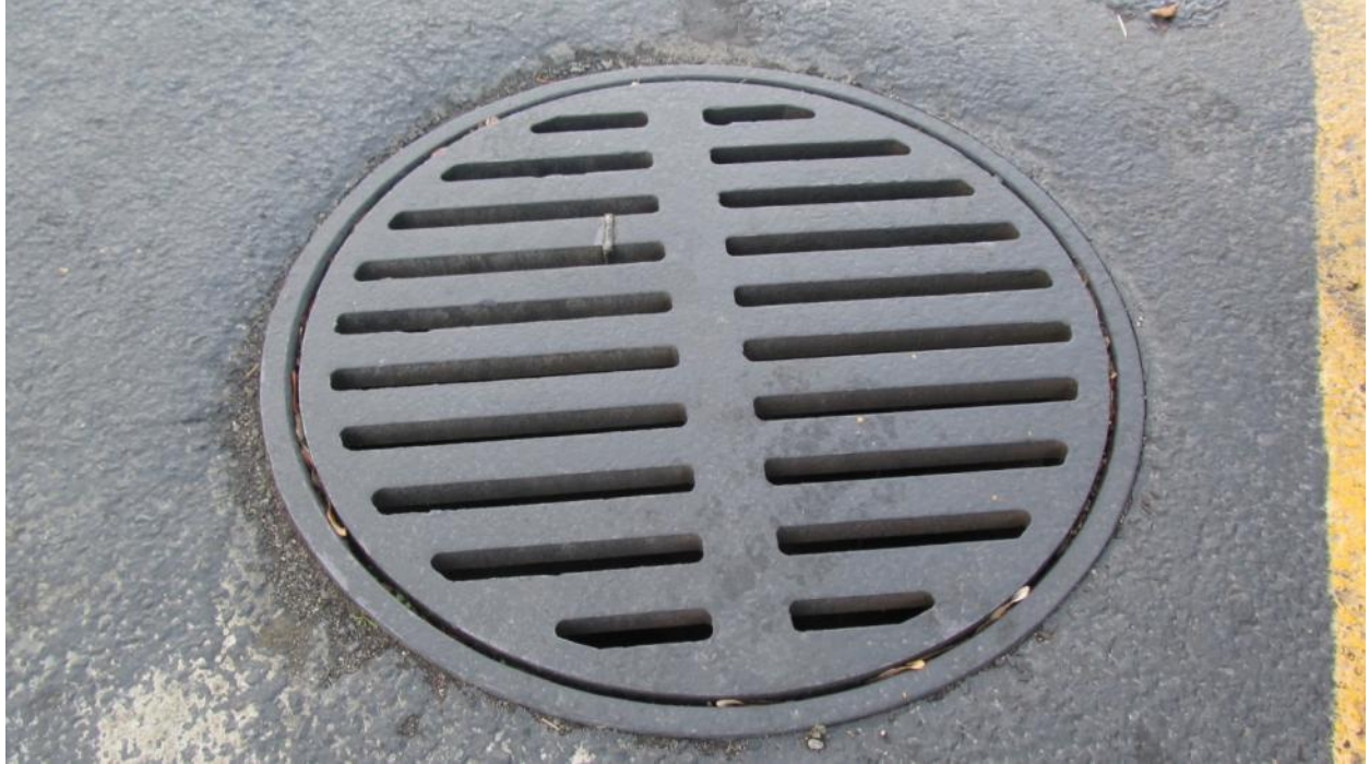
Photo 3: Dry Well with Sorbent Material - from the west
