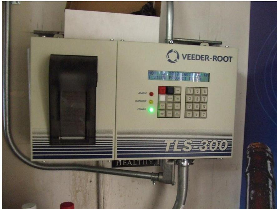
**Photo 11.** A view of the fuel monitoring system.
