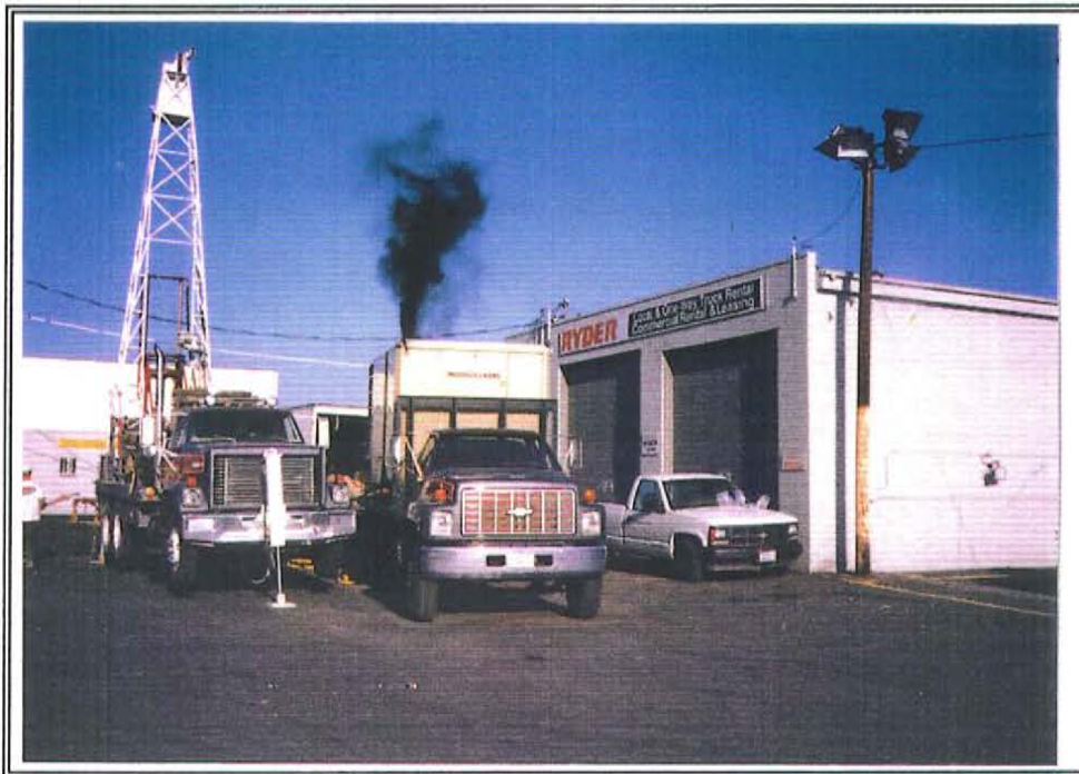
PHOTOGRAPHER: Paul Danielson DATE: 9/2/94 VIEW: Drilling MW #4 DIRECTION: Looking Northwest
