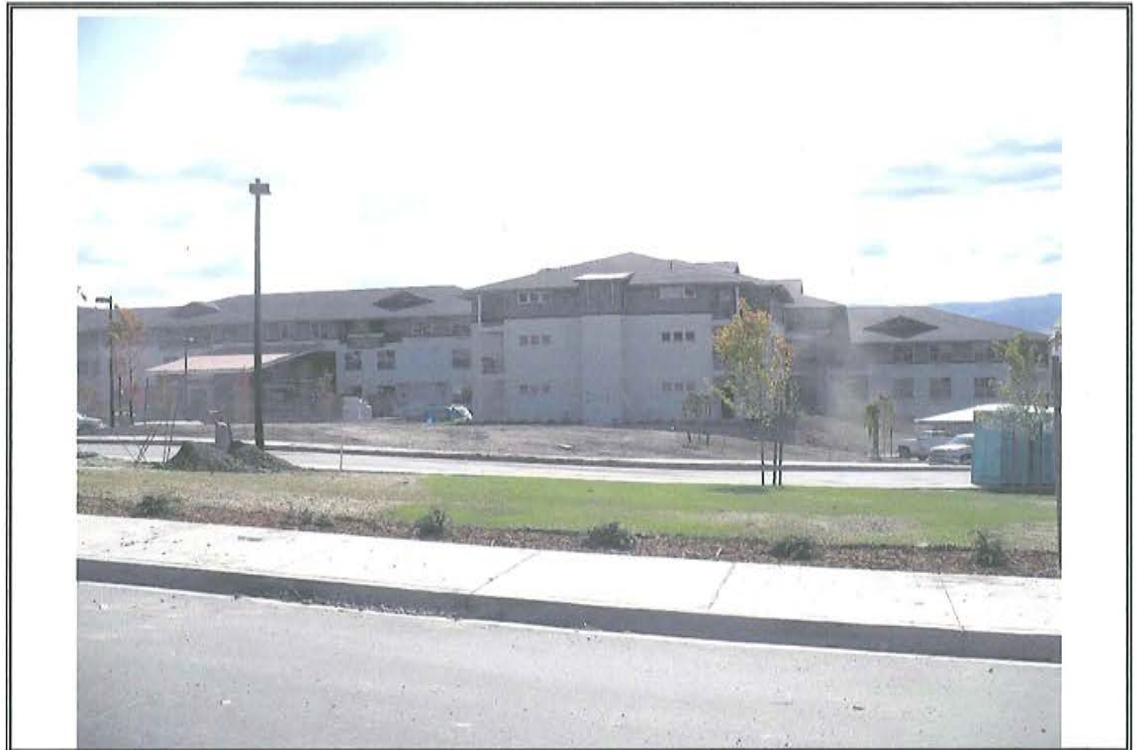
Photograph Number 17: The sod-covered area in the foreground of the photo is an area capped with a six-inch layer of clean fill and covered with sod.
