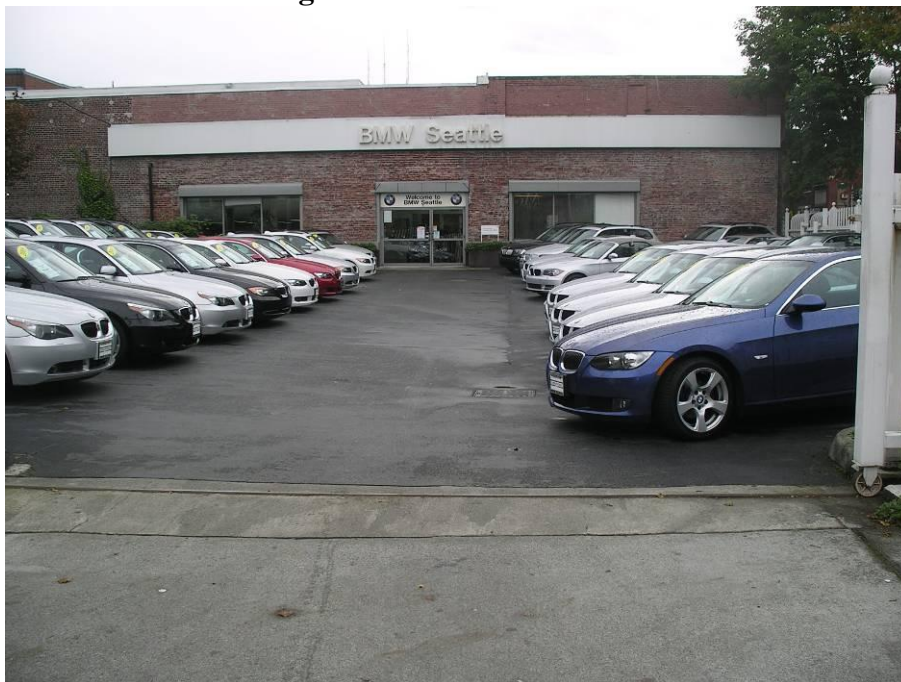
Photo 4: South Side of the Building – from the south
