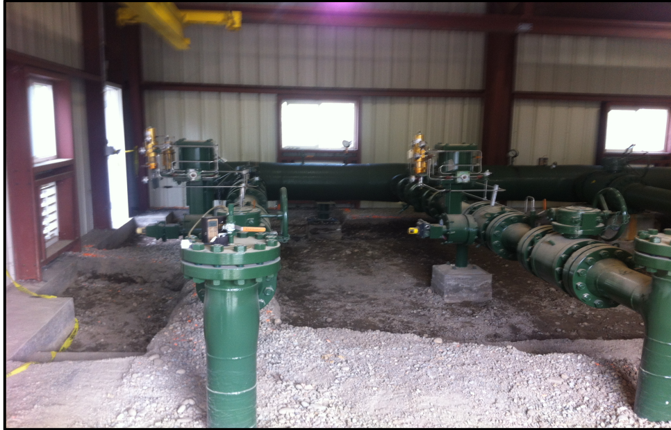
1. Looking at initial excavation.
