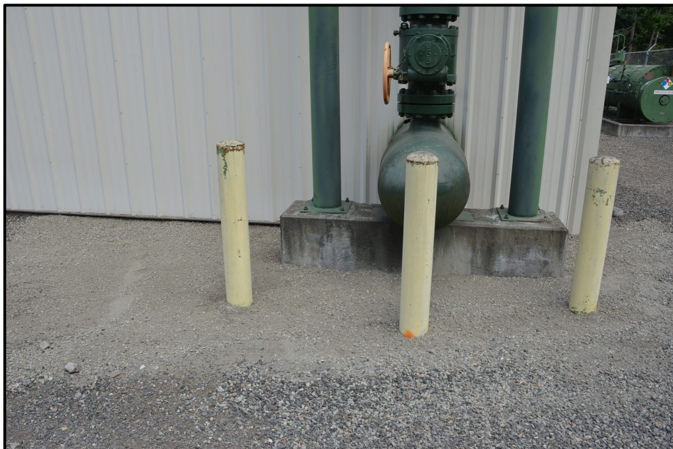
4. Looking at restored site outside building.
