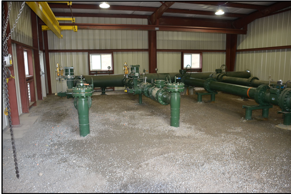
3. Looking at restored site inside building.
