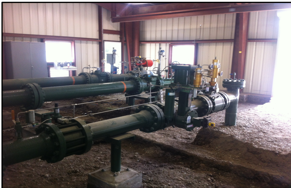
2. Looking at initial excavation.
