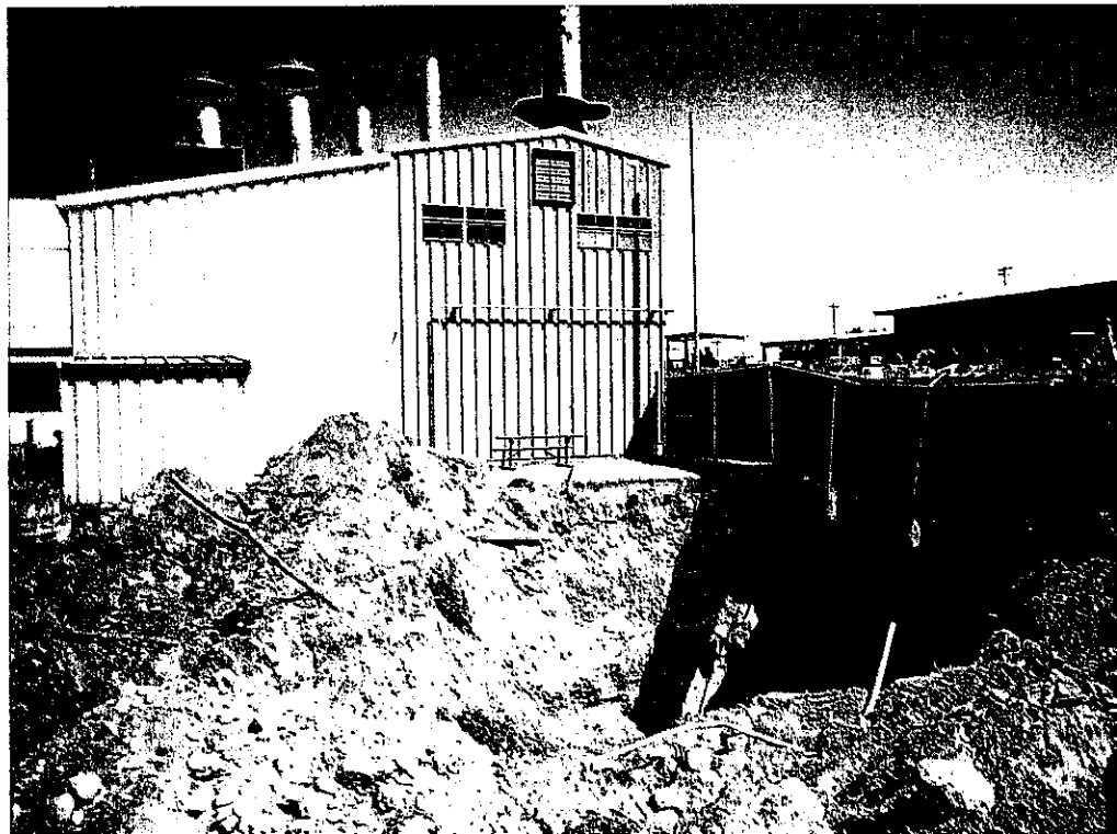
PHOTO 4: LOOKING SOUTHEAST, SHOWING INTERIM REMEDIAL ACTION CONTAMINATED SOIL REMOVAL EXCAVATION
