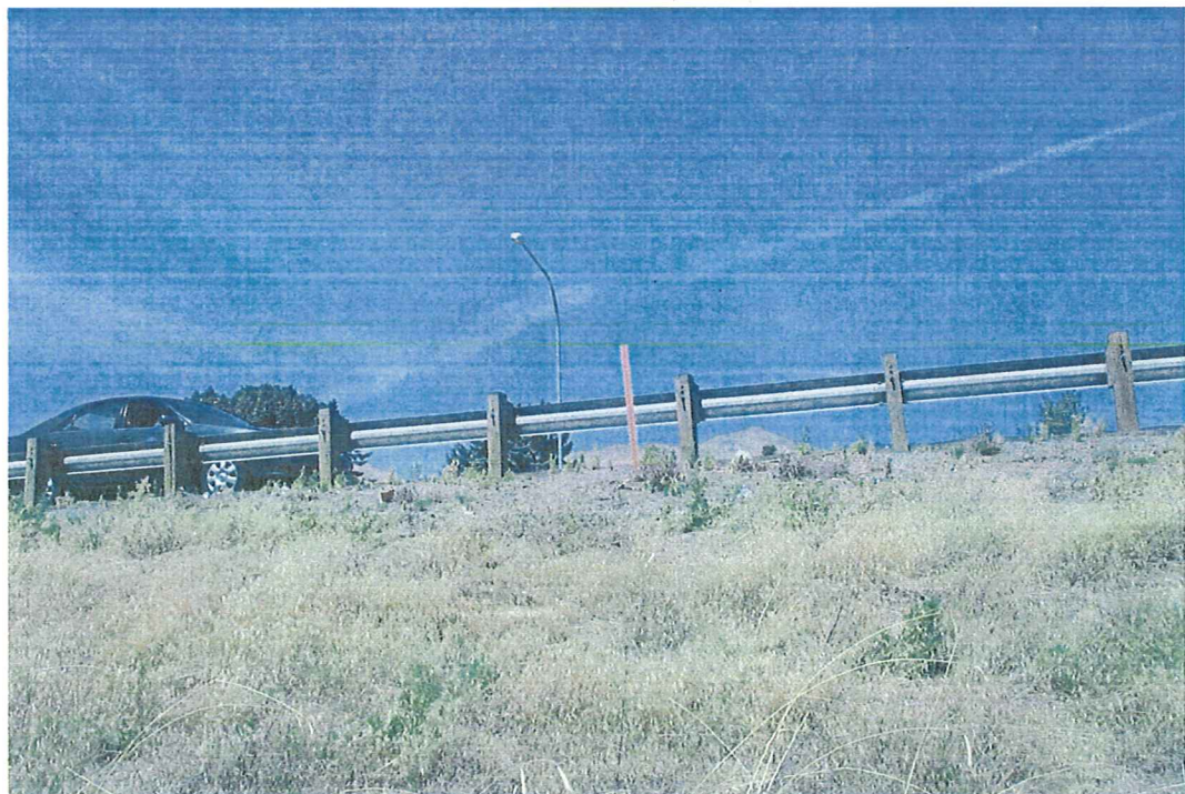
view looking up to road
