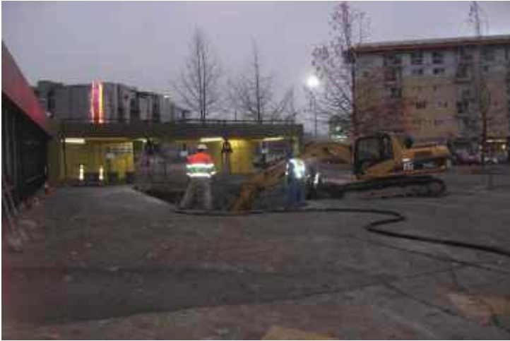
Photograph 05: Removing excavation water.
