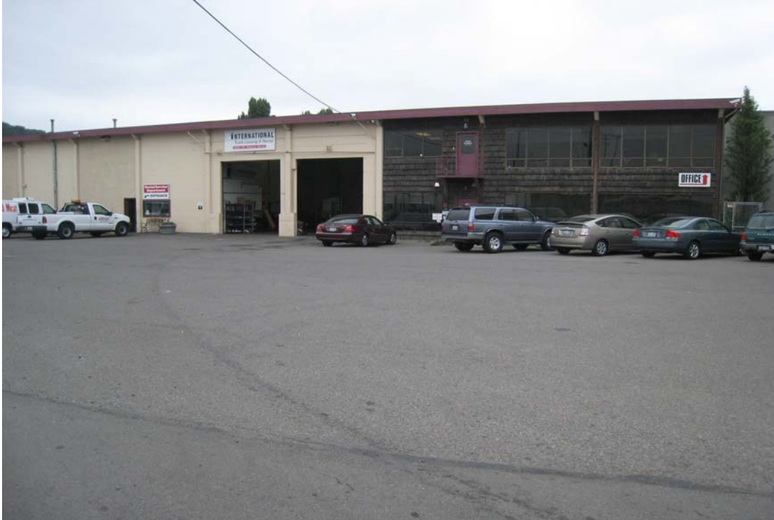
Photo 3: International Truck Leasing Building – west end, looking from the north
