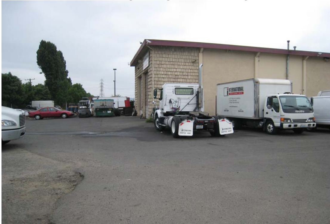
Photo 4: International Truck Leasing Building – east end, looking from the north
