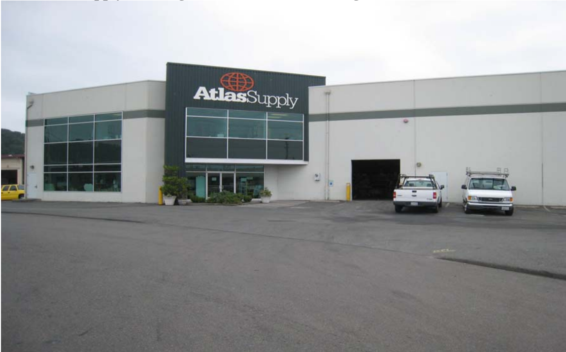
Photo 1: Atlas Supply Building, - from the north, looking southeast
